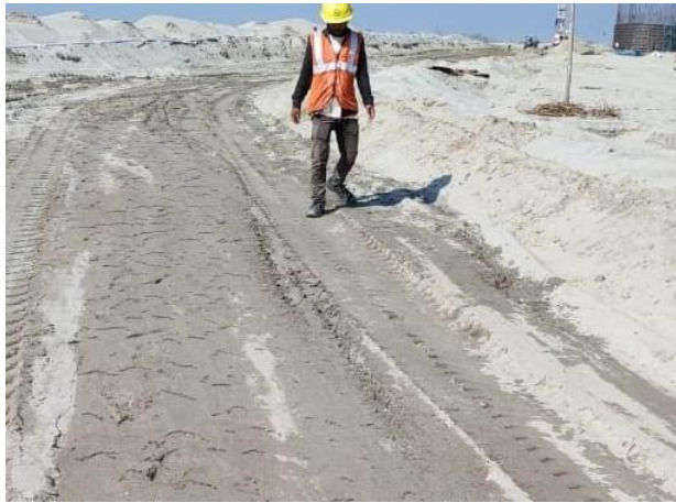
Fig. 9. The top surface after (a) four-wheel passes, (b) six-wheel passes.
