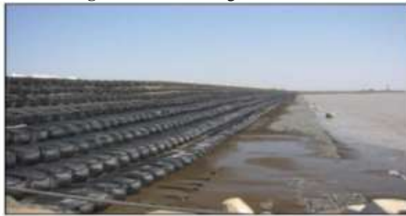
Fig.9 Reclamation of bundh using geotextile container
