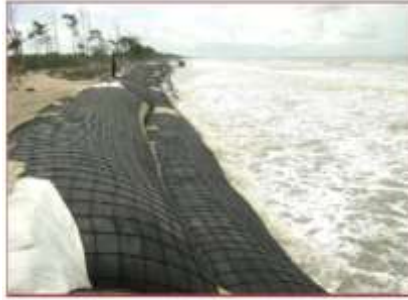
After Installation - During High Tide
