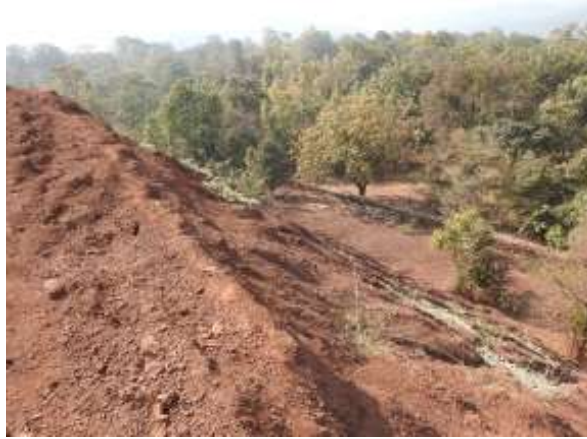
Fig. 1. Destabilized OB Dump of Slime
