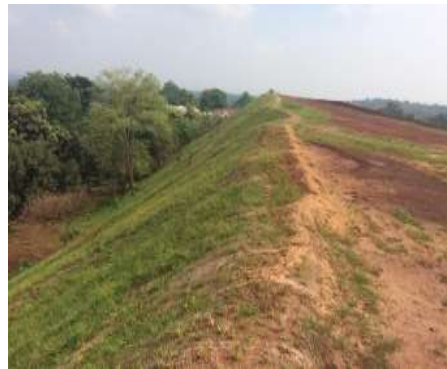
Fig.2 Laying of JGT on Slope Surface Fig.3 Stabilized OB Dump with growth of vegetation
