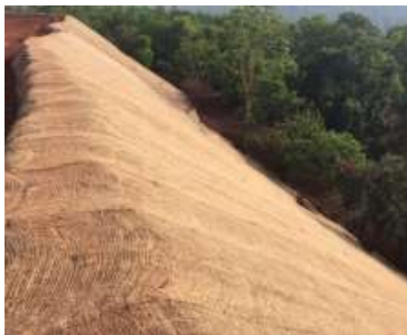
Fig.2 Laying of JGT on Slope Surface Fig.3 Stabilized OB Dump with growth of vegetation
