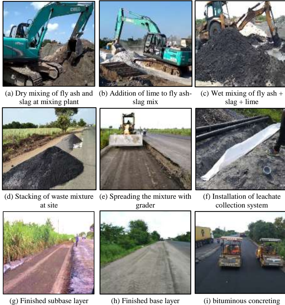
Fig. 1. Construction sequence of test sections
