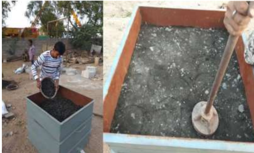
Fig 5. Preparation of base course layer
