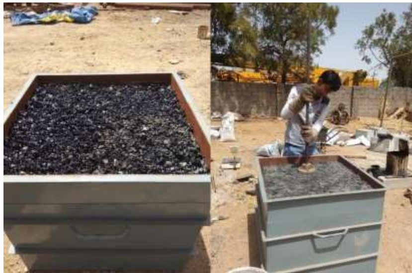
Fig 6. Preparation of Wearing course
