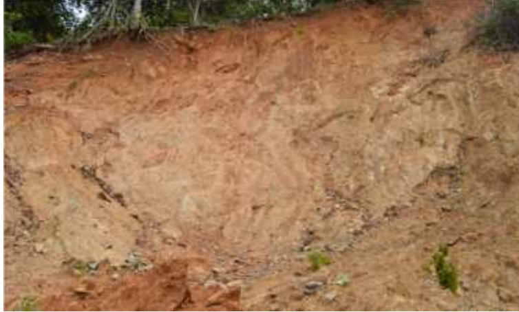
Fig. 2. Lithology at the site of failure at Kuranjeri
