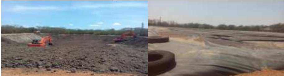
Fig. 1. Preparation of slope for leachate pond and placing of geo membrane at slope
