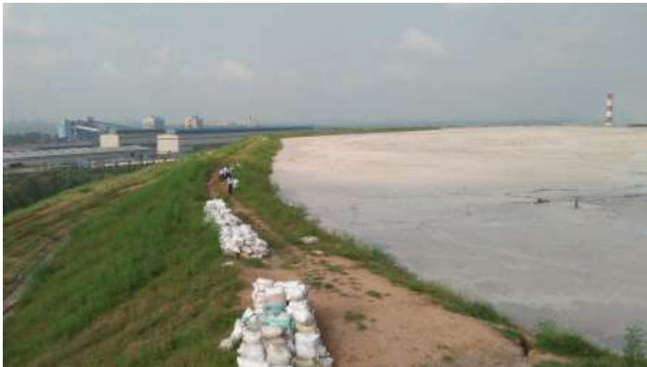
Fig. 13. View of Ash Pond Side above Gabion Wall
