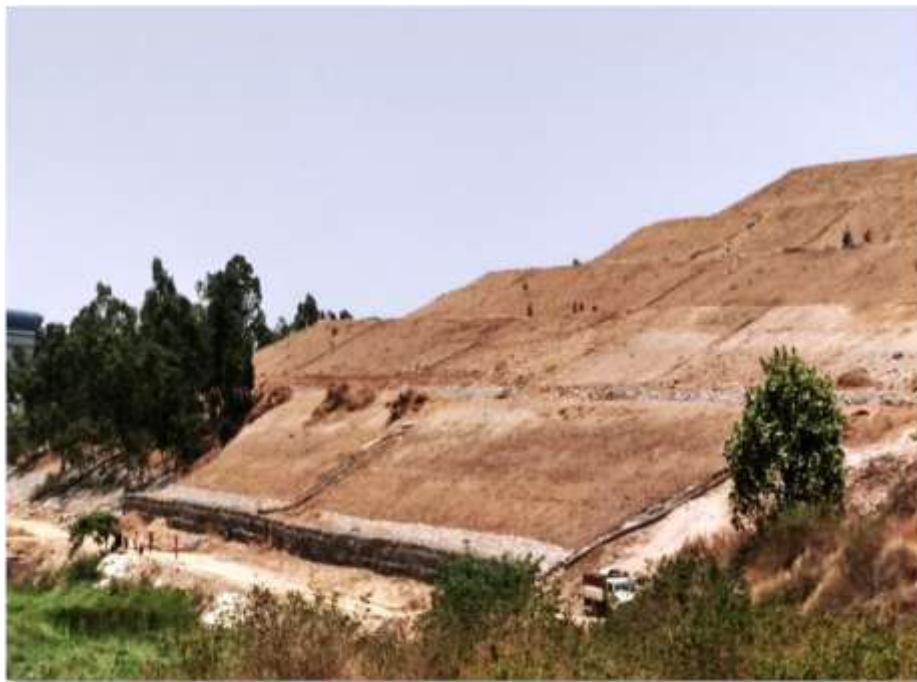
Fig. 11. Gabion Wall and Slope Profiling during Retrofitting at Subsidence Stretch
