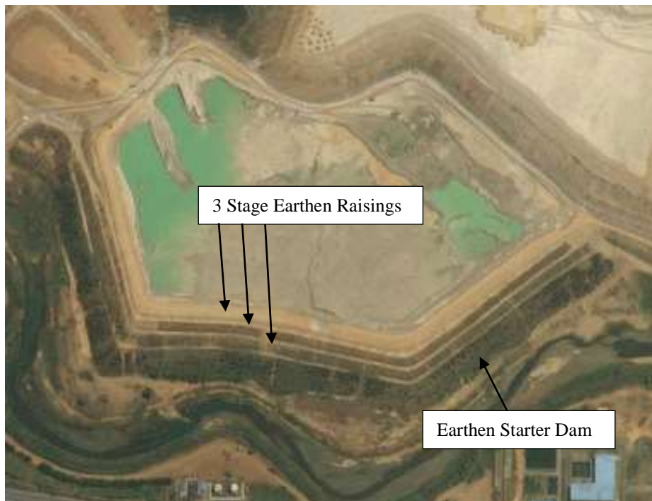
Fig.1. Ash Pond after 3rd Raising (Source Bing Satellite Image)
