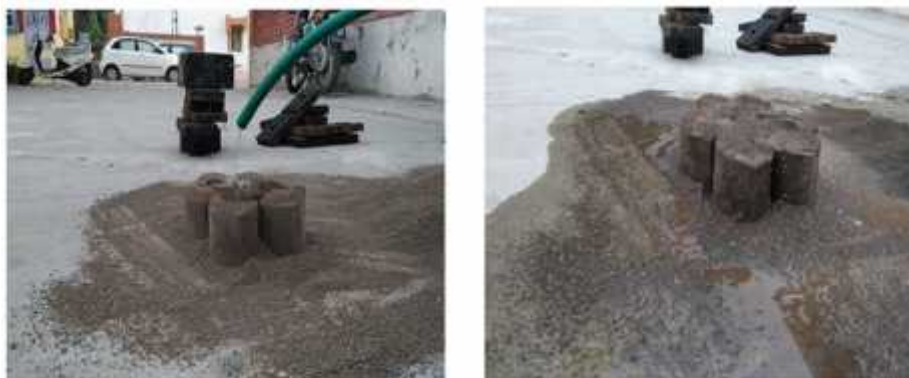
Fig 5. Drainage test using Geo-cell
