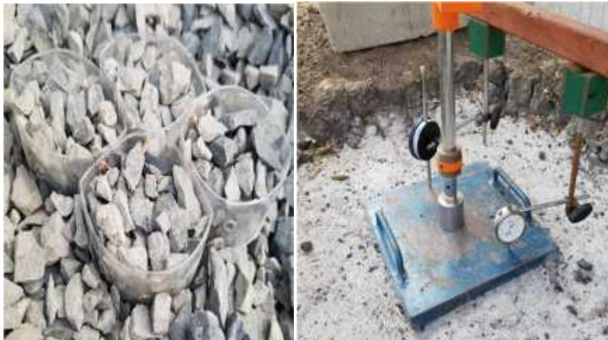
Fig 8. Closed views of Geocell and plates for plate load test
