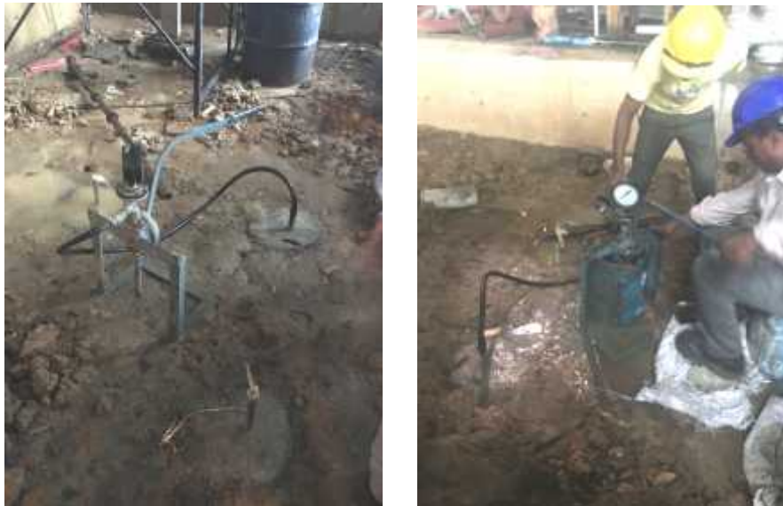
Fig.5. Trial grouting in progress
