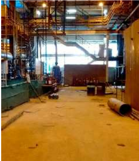
Fig.9. Holes cored in between equipment for grouting Fig. 10. Schematic of grout hole
