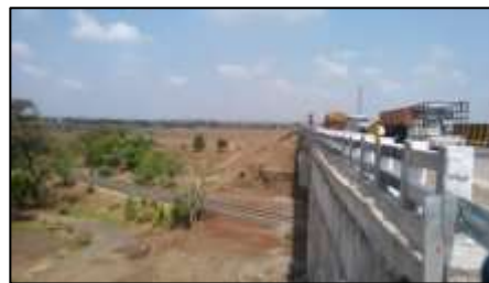
Photograph 5 : Railway Over Bridge (ROB)
