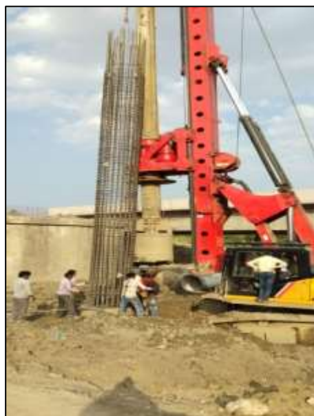
Photograph 1 : Piling Rig deployed in Site
