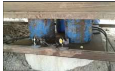
Photograph 3 : Jacks and Dial Gauges in Load Test
