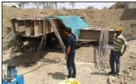
Photograph 2 : Set-up of Vertical Pile Load Test
