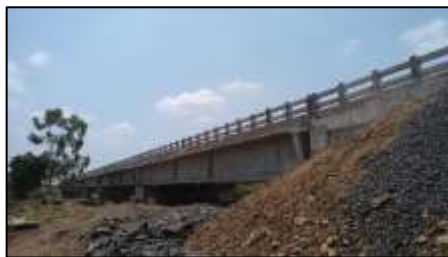
Photograph 4 : Major River Bridge
