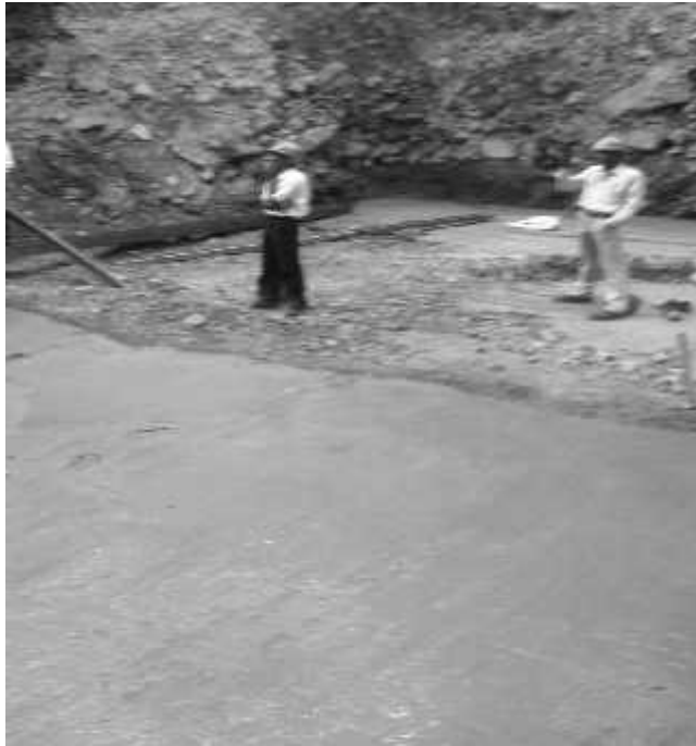
Fig.5: Plum Concrete Laid in Part Area
