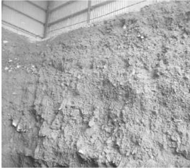
Fig.4 : Mortar Application on Slope
