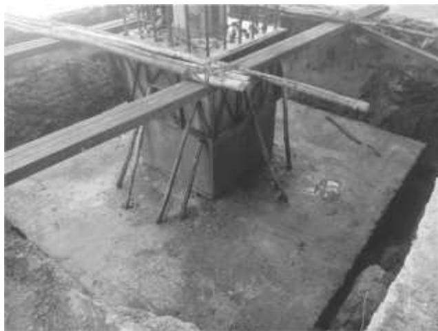
Fig. 6. Site photos showing footing after concreting
