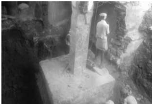
Fig. 4. Site Photos showing existing footing and underpinning before concreting
