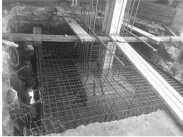
Fig. 5. Site Photos showing underpinning before concreting
