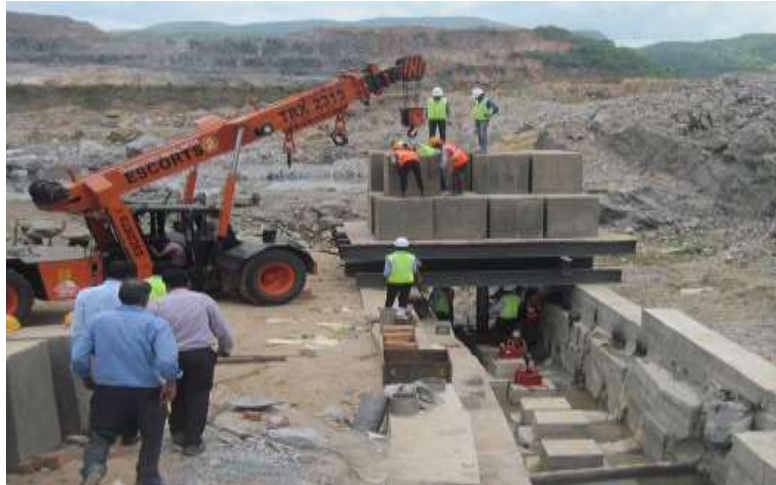
Fig. 4. Photograph of open trench showing Kent-ledge loading arrangement [10]
