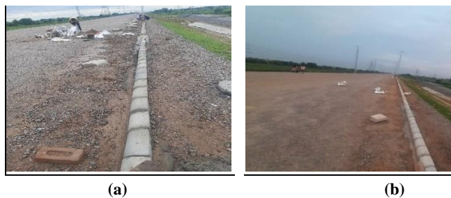
Fig. 5 (a)-(b). Kerbs with chute drains at the top of the formation.
