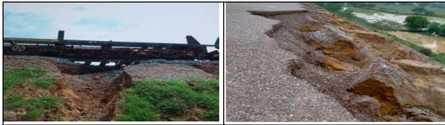
(a) Rain-cut in track platform
