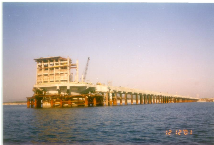
Fig.11. Completed view of the Approach jetty and Intake
