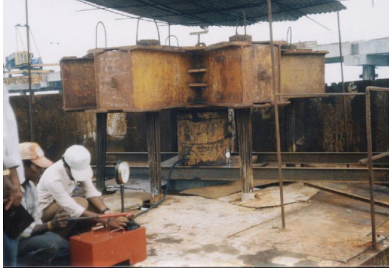
Fig.8 . Test arrangement of simulated initial pile load test
