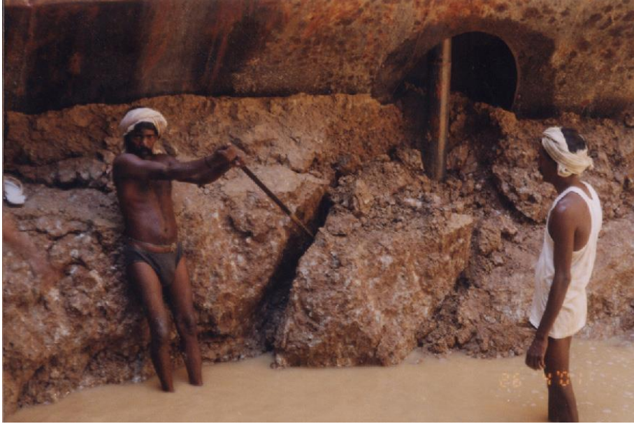
Fig.6. Rocky strata at Intake well location
