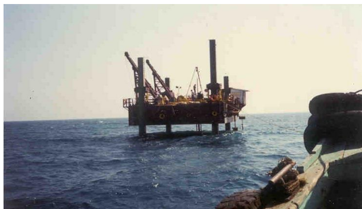
Fig. 3. Hydraulic rig for geotechnical investigation on Jack up platform .
