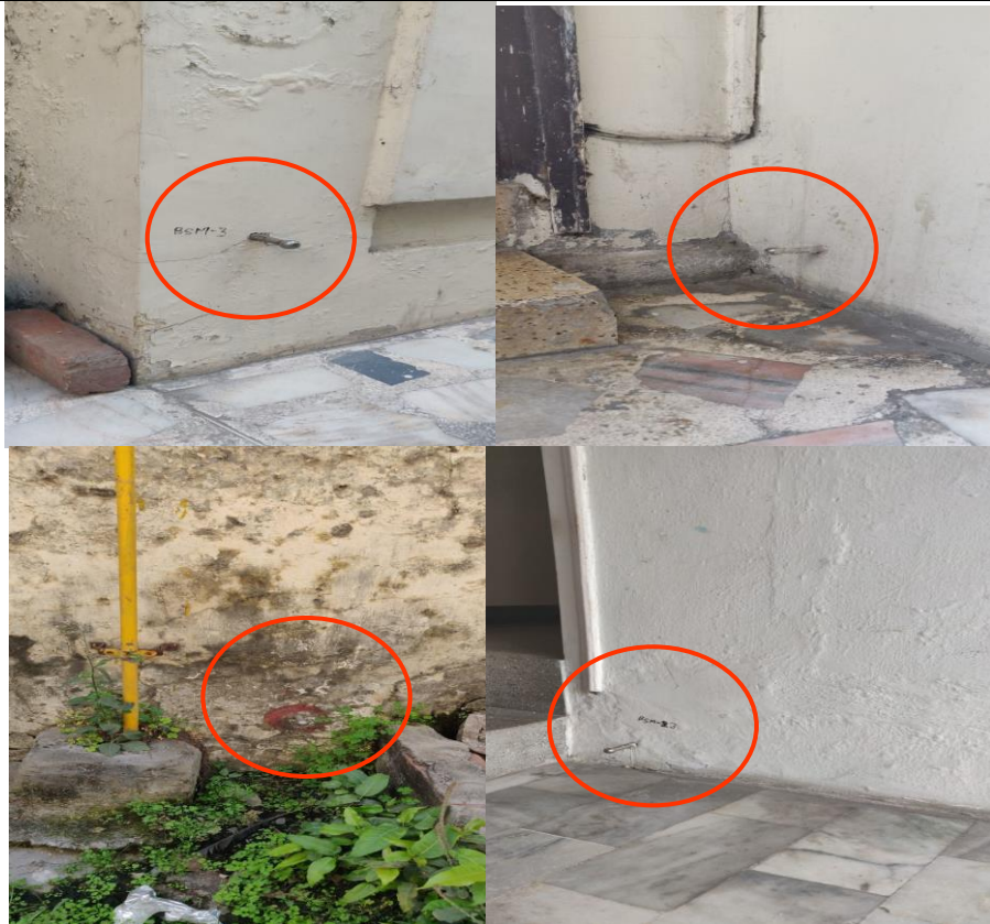
Fig. 5. Building Settlement Marker Locations
