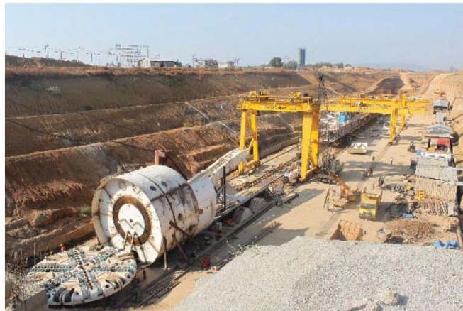
Fig. 2. Onsite assembly of TBM
