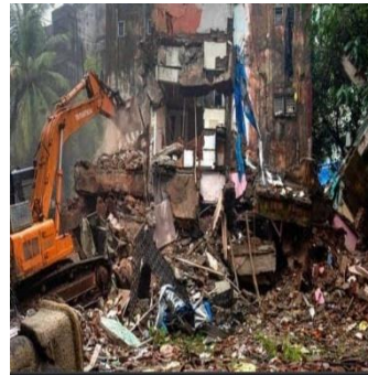
Fig.4. Demolition of the building
