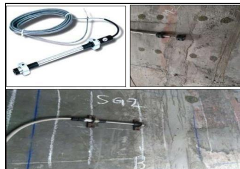
Fig. 5. Strain Gauge and Crack Meter Measurement
