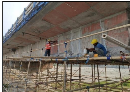
Fig.15. Grouting application procedure
