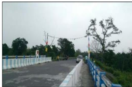
Fig. 2. Upper view of Dima bridge
