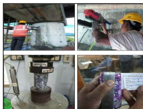
Fig. 8. Drilling of Concrete Cores
