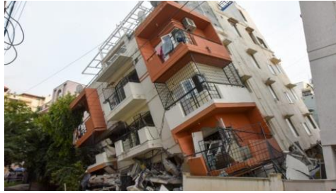
Fig.1. Failed structure at Kasturinagar.
