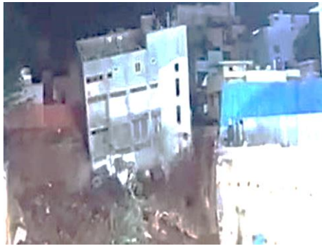
Fig.6. Failed structures at Gandhinagar.
