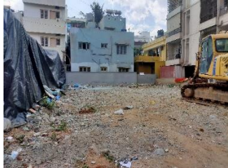
Fig.3. Kasturinagar site after demolition
