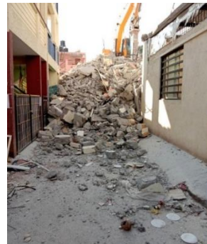
Fig.6. Demolition of the building
