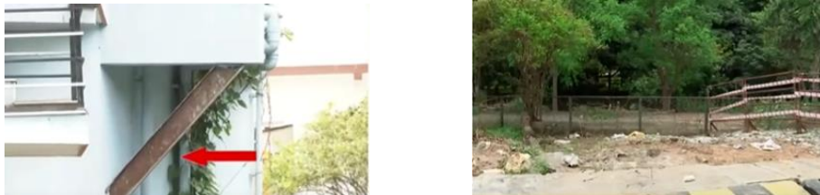
Fig.9. Temporary support to the building at Poornachandra layout
