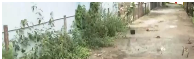
Fig.8. Building constructed adjacent to the storm drain side wall
