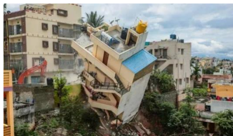
Fig.1. Building falling back due to foundation failure
