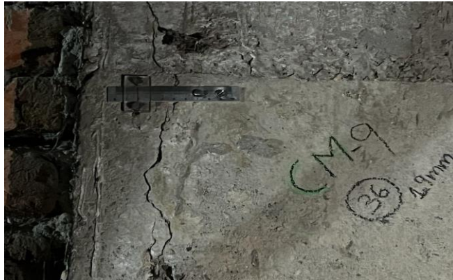
Fig.11. Placing of crack meter for monitoring crack variations after blast
