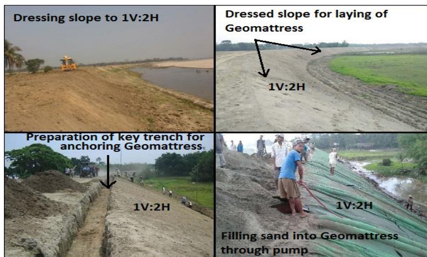
Fig. 7. Installation of Geotextile mattress at various stages
