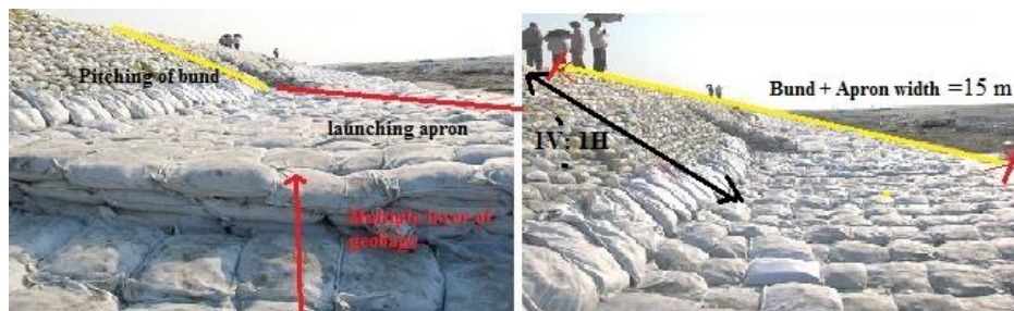
Fig. 10. Pitching of Tie-bund and launching apron
