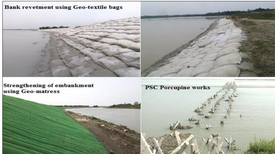
Fig. 4. Implementation of Geotextile bags, Geo-mattress and PSC Porcupine works
