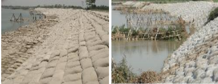
Fig. 13. Implementation of geotextile bags in revetment and launching apron
