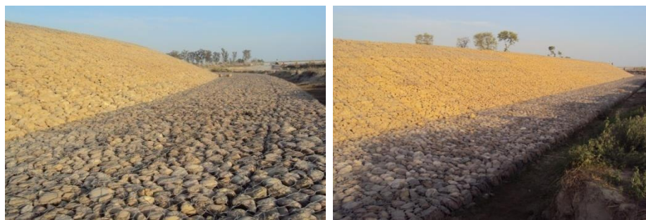
Fig. 6. Completed embankment in Phase-II
