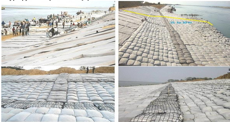
Fig. 2. Placement of the filter media, Geobags & Polypropylene Rope Gabions
