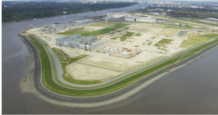
Fig. 6. Hamburg air-plane dockyard extension site (Huesker Synthetic GmbH [28])
