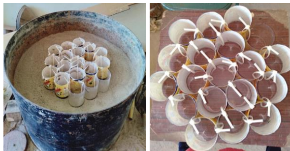
Fig. 2. Preparation of geocell reinforced sand bed
