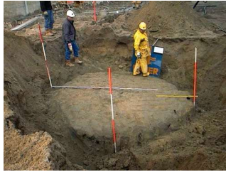
Fig. 5. Jet grout columns with 4.35 m diameter in clean sand
