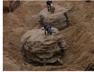
Fig. 5. Jet grout columns with 4.35 m diameter in clean sand
