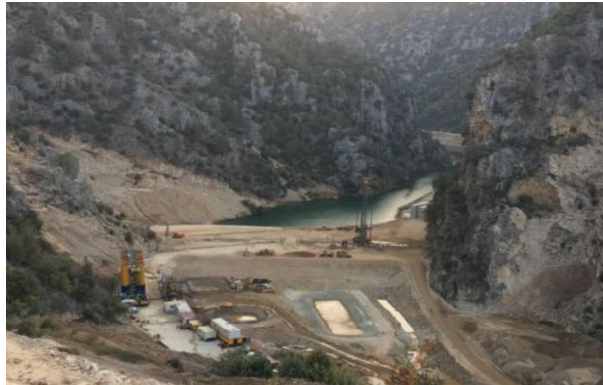
Fig. 3. Execution of cut-off wall at upstream cofferdam
