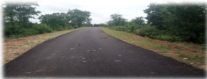
Fig.3. Road constructed by treating with terrazyme ( Source: info@avijeetagencies.com )
