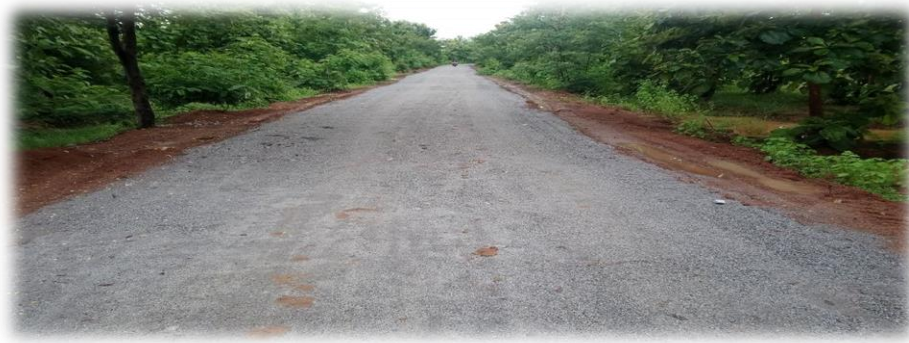
Fig. 4. Terrazyme treated road condition after one monsoon season
