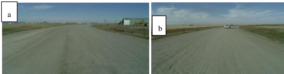
Fig. 7. a) Improved surface, b) Reduction in dust
