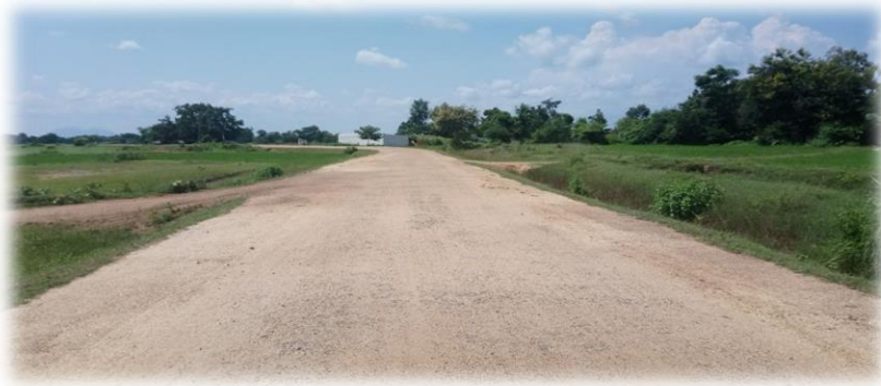
Fig. 2. Road treated with terrazyme
