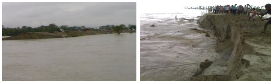
Fig. 1. Breach and Flood problem before execution of Geo Dyke
