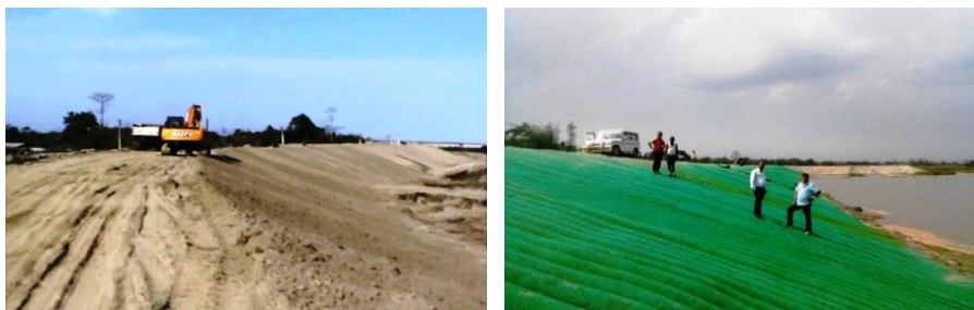
Fig. 6. Installation of Geotubular mattress
