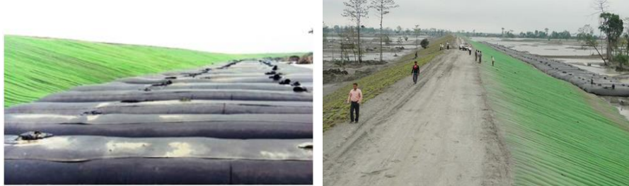
Fig. 5. Installation of Geotube as scour apron at Matmara geo-dyke
