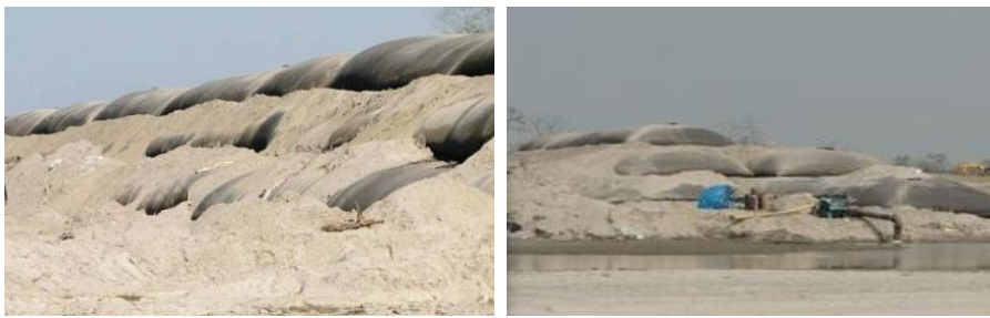
Fig. 3. Installation of geotubes (1:2:3) as core of the embankment
