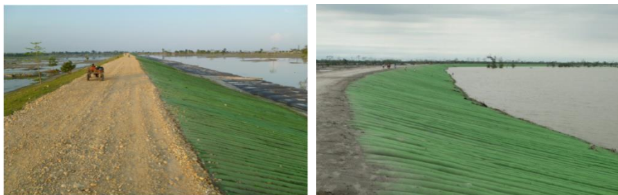
Fig. 4. Installation of Geotubular mattress as revetment
