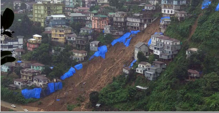
Fig. 3. Affected area above National Highway
