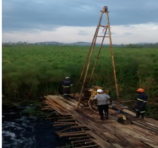
Fig.1. Geotechnical Investigation in Swamp
