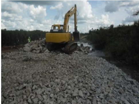
Fig. 4. Compaction of rocky material in Swamp
