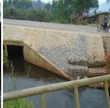
Fig.5. Typical RCC Box Culvert in Swamp
