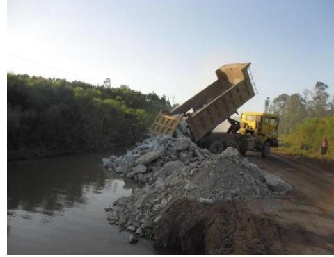
Fig.3. End tipping work of rocky material in Swamp
