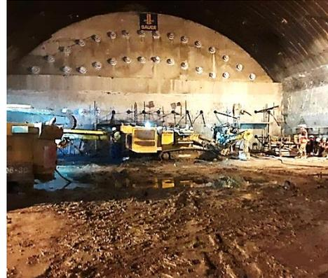
Fig. 12. General view and details of anchor heads
