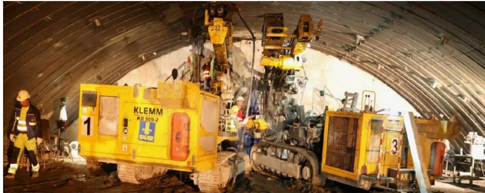
Fig. 7. Two Klemm KR 909 rigs working in narrow space inside the cavern
