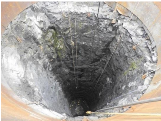
Fig. 5. Excavation of delivery main vertical shaft-01 under progress.
