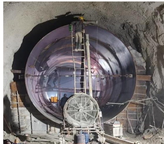
Fig. 4. Steel lining work of delivery main tunnel-2 horizontal portion under progress.
