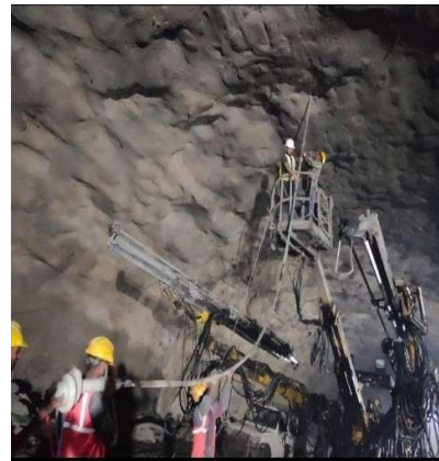
Fig 12. MPBEx installation
