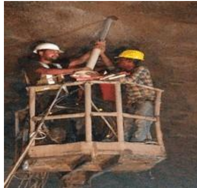
Fig 10. MPBEx installation
