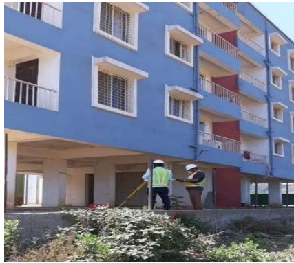
Fig 9. Settlement observations in building
