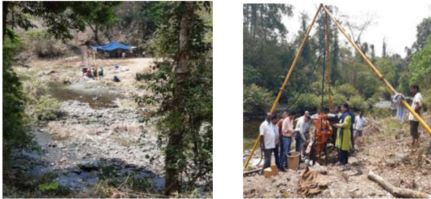
Fig 2 Drilling work in progress at dam site
