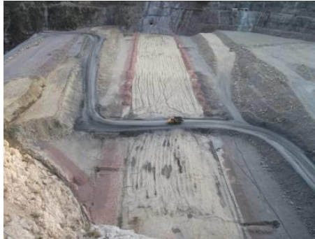
Fig. 6. The crossing road over the filter zone
