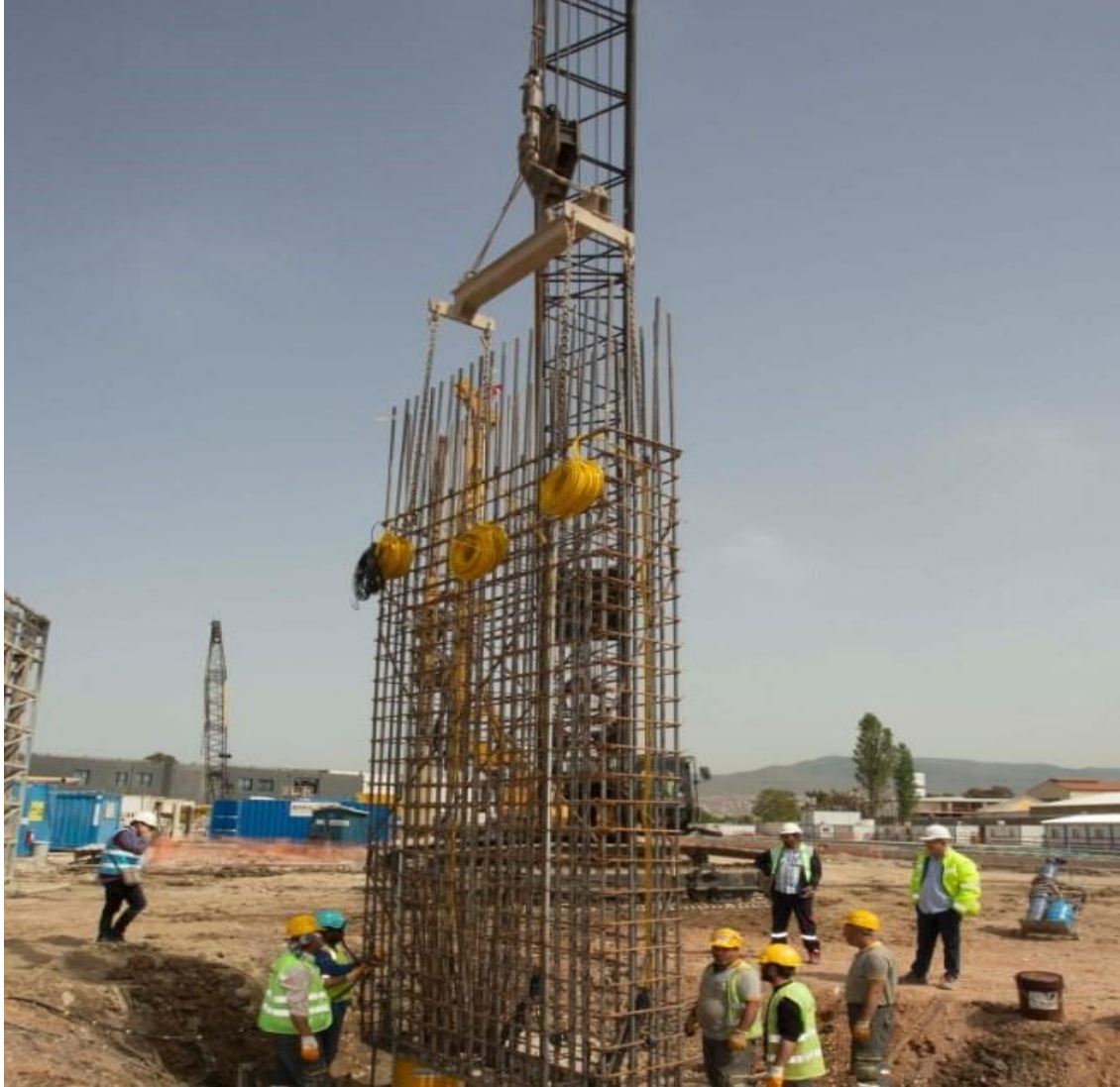
Fig.1. Barrette installation
