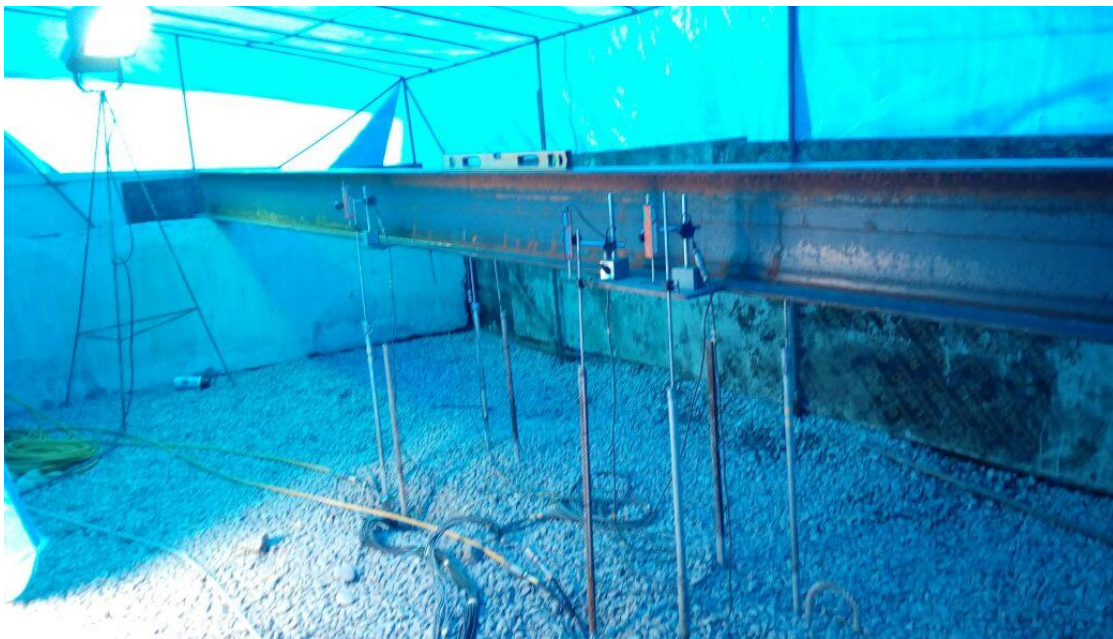
Fig. 2. Barrette load test set up
