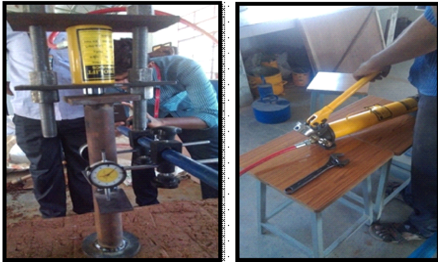
Fig. 1b. Total test arrangement of the footing placed on soil bed along with hydraulic jack and dial gauges
