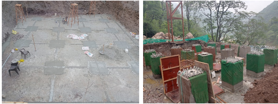
Fig. 12. Foundation construction in progress
