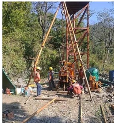
Fig. 8. Borehole Drilling in Progress
