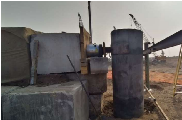
Fig. 4. Lateral Load Test Set Up
