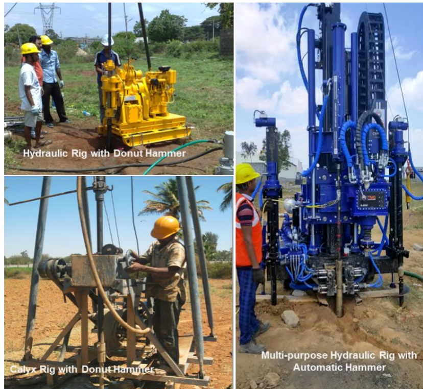
Fig 1. Different Geotechnical Rigs with different Hammers
