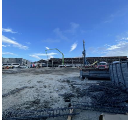
Fig.7. Parking garage site
