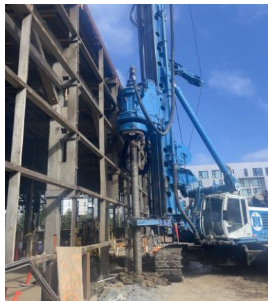
Fig.2. DDC installation at the site
