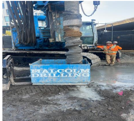
Fig.12. Recalibration of Rig grout factor
