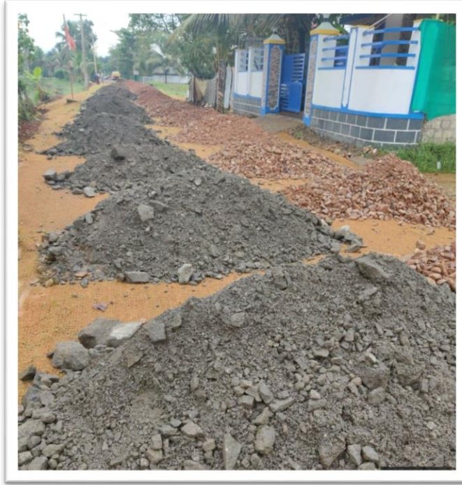
Preparation of Sub base
