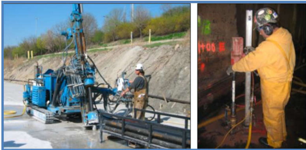
Figure 7.2. Track-mounted and hand-held high-speed rotary drills.
