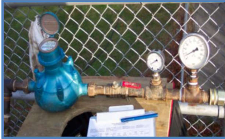
Figure 7.8. Manually read mechanical water meter and pressure gauges for pressure testing.
