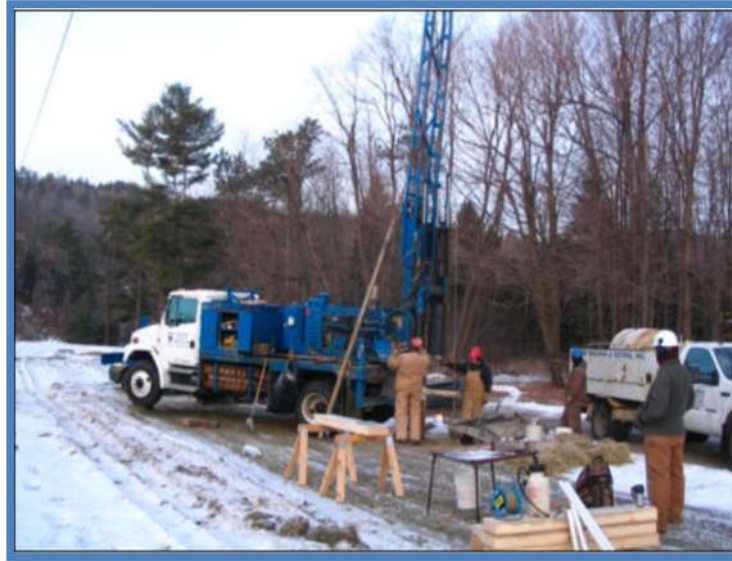
Figure 7.1. Truck-mounted high-speed rotary drill rig. (Courtesy of Gannett Fleming)
