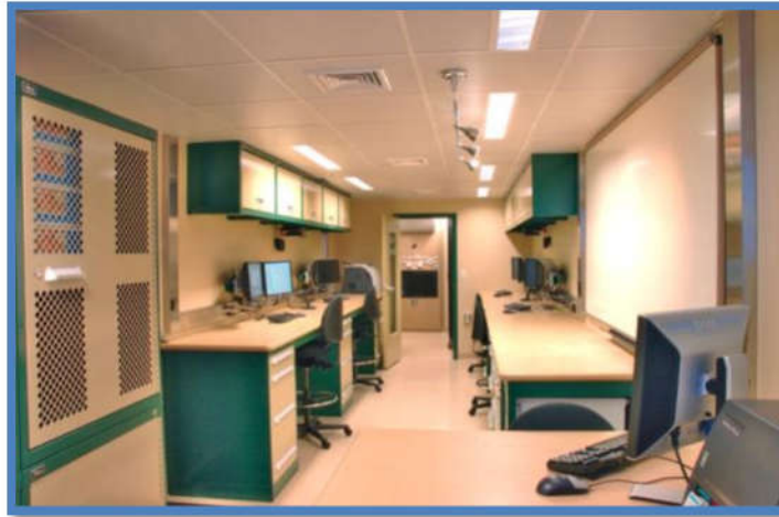
Figure 8.1. Centralized automated system for real-time processing and display for actively monitoring and controlling injections. (Courtesy of Gannett Fleming)
