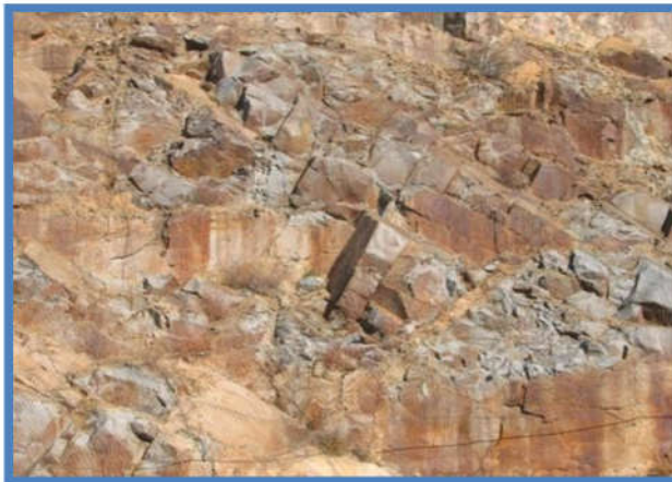
Photo 4-5: Abutment area of Olivenhain Dam, CA.
