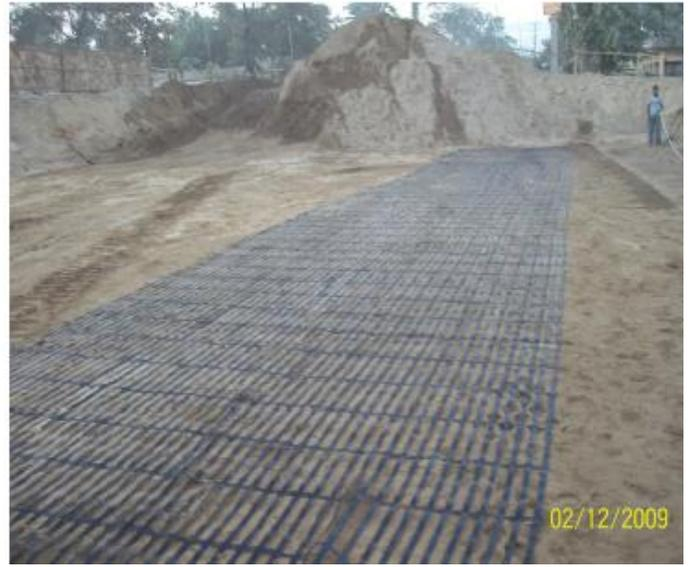
**Fig-5: Installed high strength uni-axial Geogrid (basal reinforcement)**
