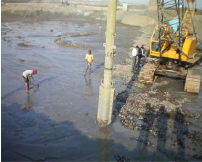
Photo 1 Installation of stone column
