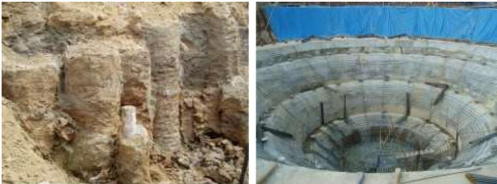
**Figure 20: Typical exposed DSM and Structure after DSM installation**
