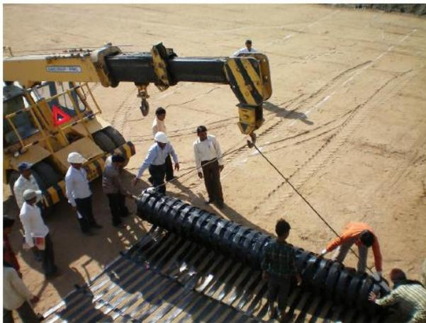
Photo 3 Laying of High strength uniaxial Geogrid
