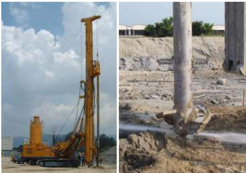
**Figure 5: Wet DSM machine & Ejection of the binder (wet form) from the machine**
