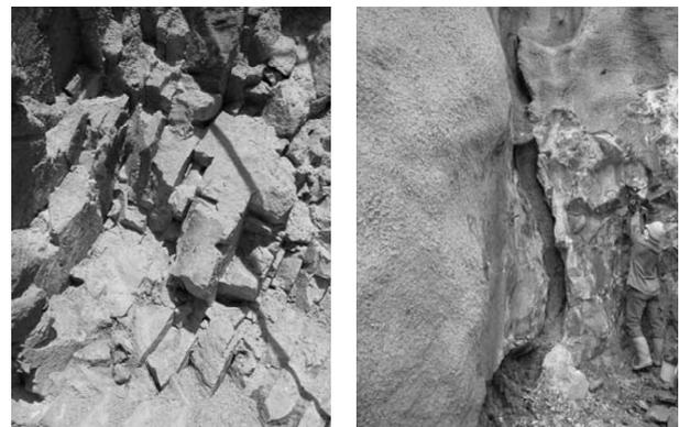
Figure 11 Rock Fissures where Water may Ingress into Excavation
