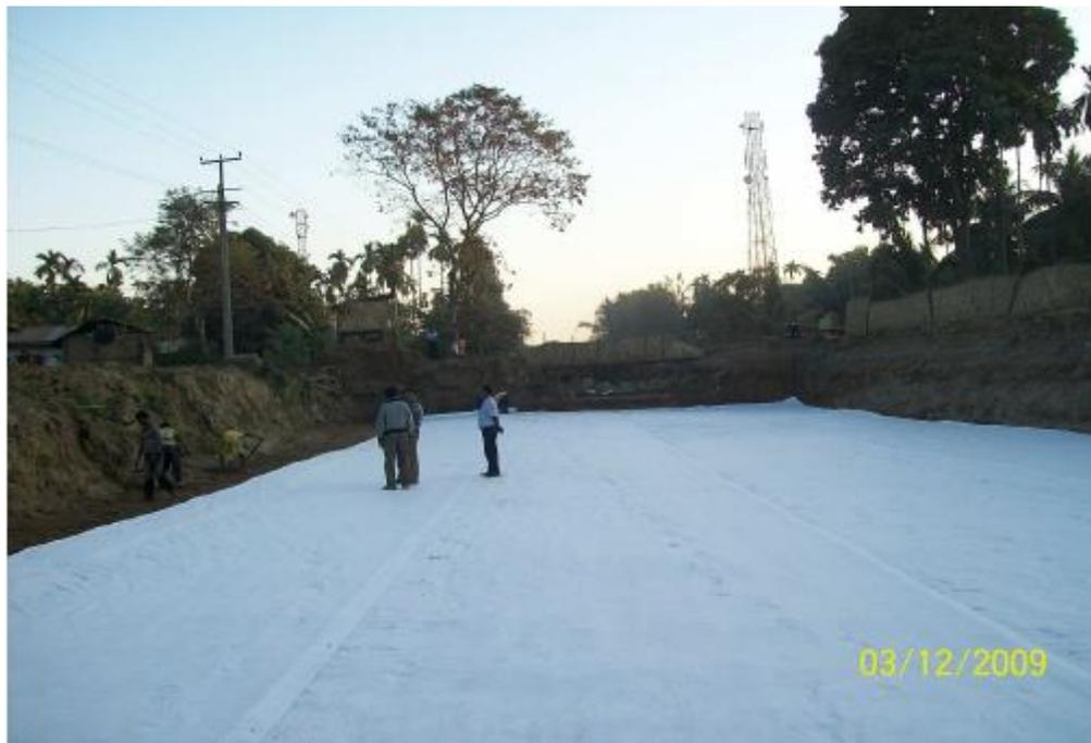
**Fig-2: Installation of Geotextile**
