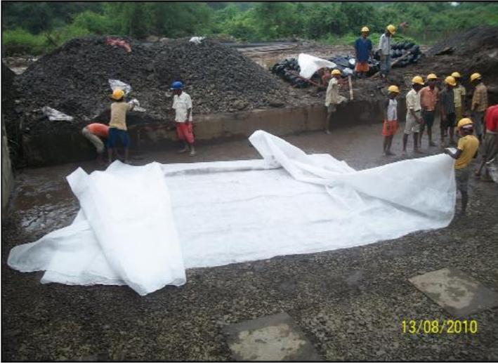
**Fig-2: Laying of Geotextile over Pile caps**
