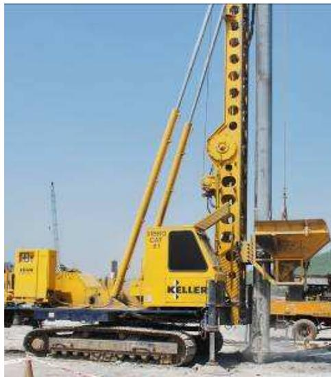
**Fig. 2** A typical Vibrocat unit
