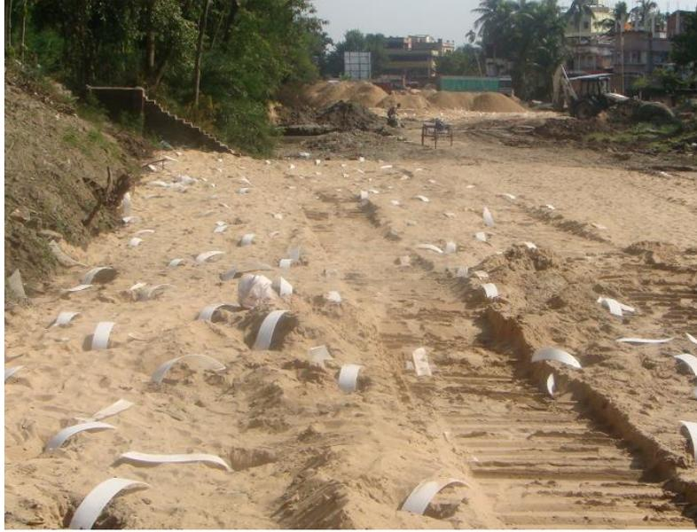
**Fig-1: Installed PVD's**
