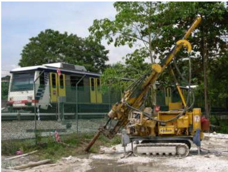
**Figure 23: Drilling and grouting beneath rail track**
