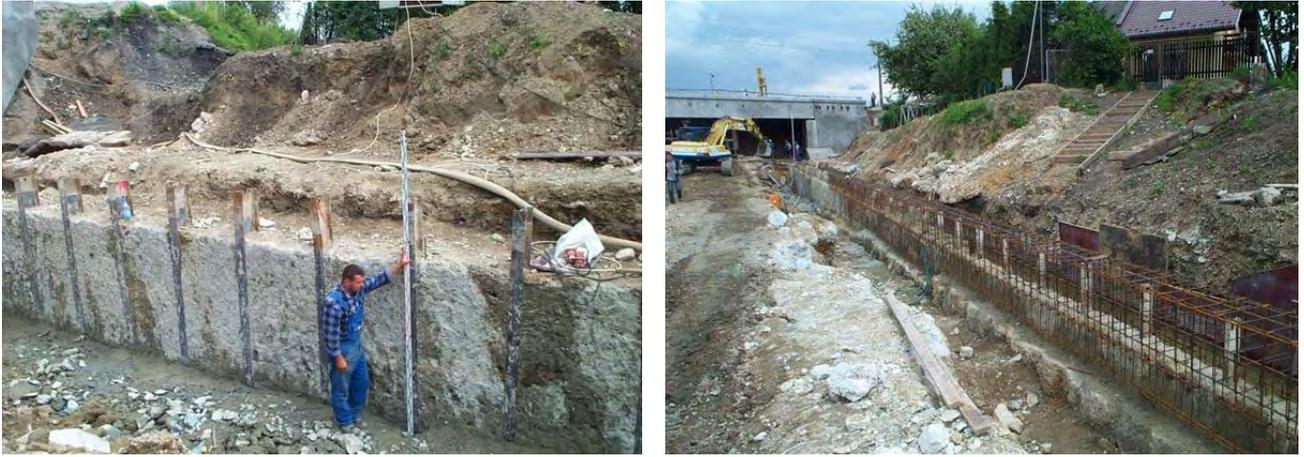
Figure 8. Permanent soil mixing retention wall with embedded steel H-beams and concrete facing (Oświęcim, Poland).
