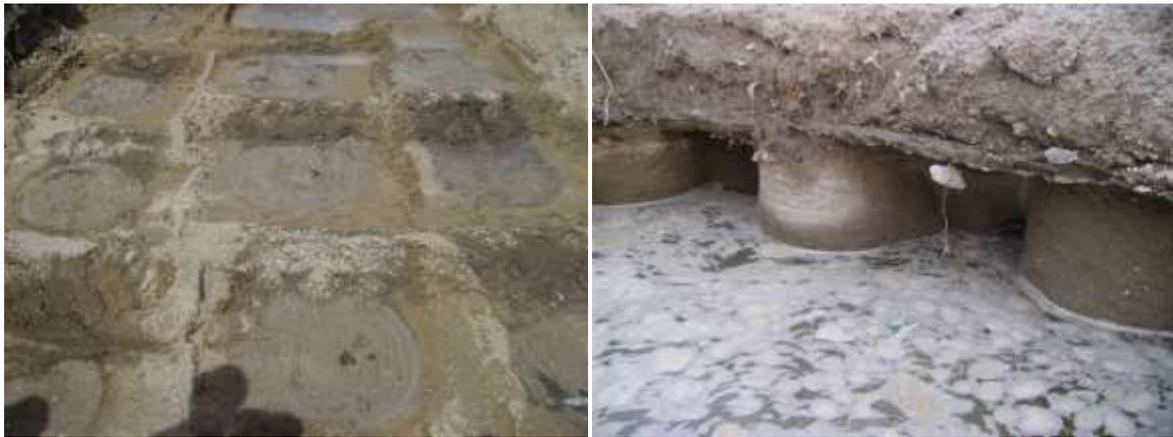
Figure 14: Visual examination of exposed columns by means of excavation
