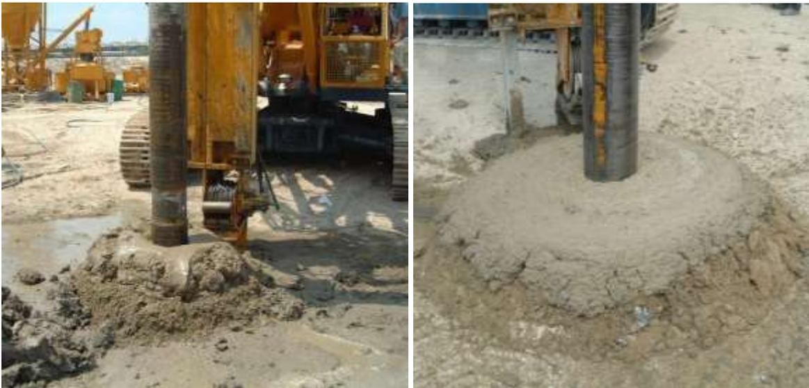
**Figure 6: Mixing operations in Wet DSM process**
