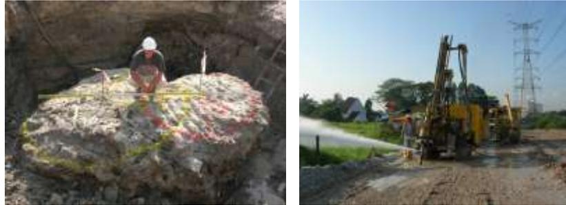
Figure 5. Exposed trial Jet Grout columns (left) and execution of working columns (right).
