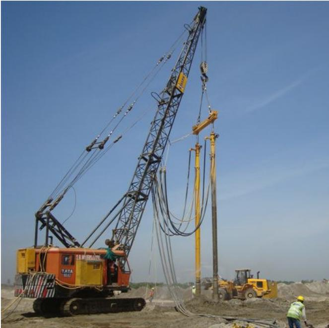
Fig. 6 Twin Vibrators in action.
