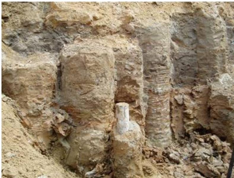
*Fig. 17 Typical exposed DSM columns during excavation*
