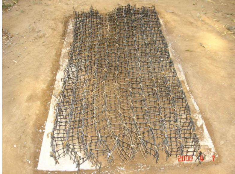
**Figure 32.** Geocell layer prepared at the site
