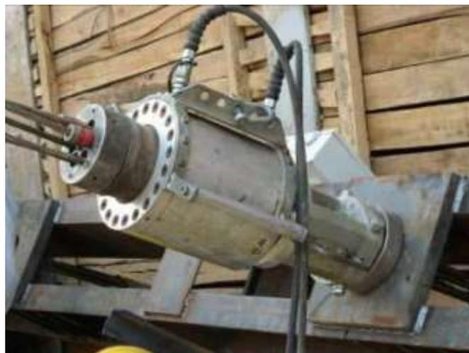
**Fig. 7:** Pre-stressing using 100T capacity multi strand jack
