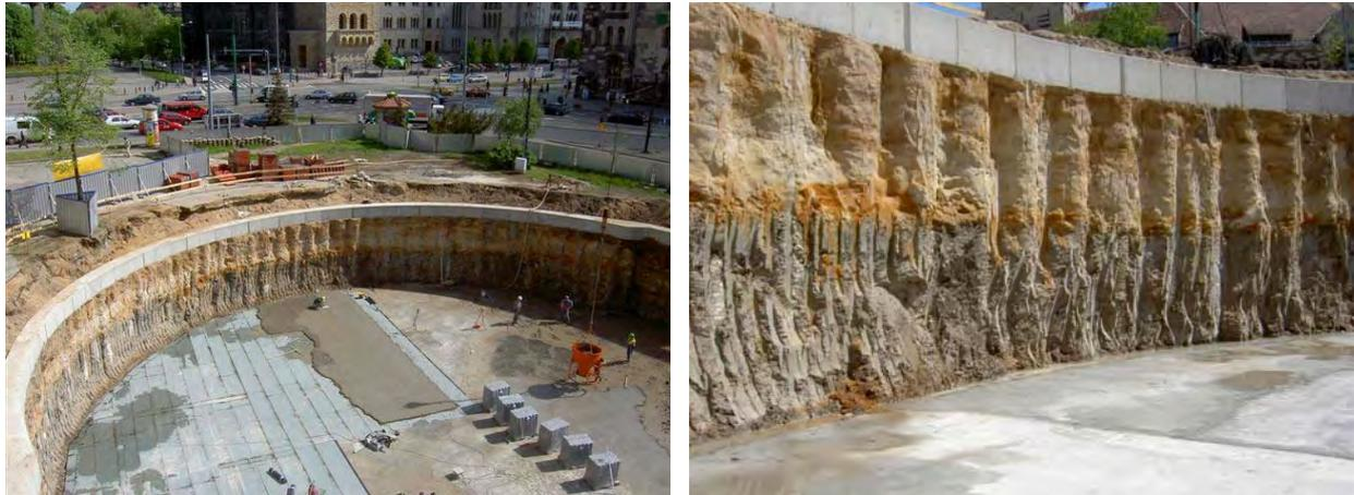
Figure 7. Temporary SM wall with embedded steel H-beams for excavation support (Music Academy, Poznań, Poland).
