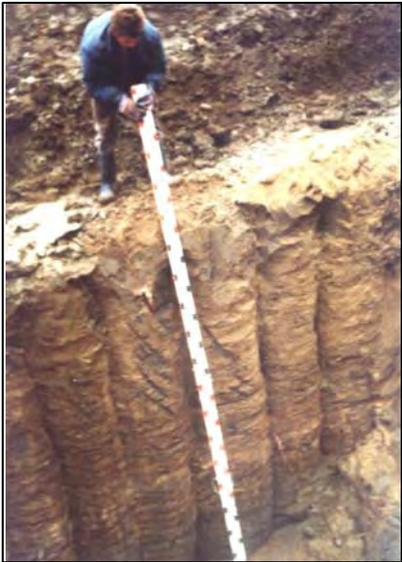
Figure 2. Soil mixing cut-off wall to intercept seepage flow paths under river bank embankment (The Vistula river near Tarnobrzeg, Poland).
