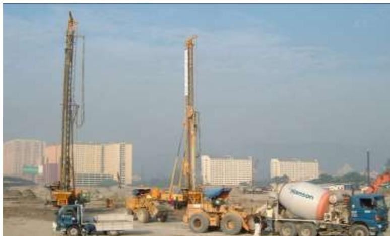
Figure 11. Picture showing execution of VCC.
