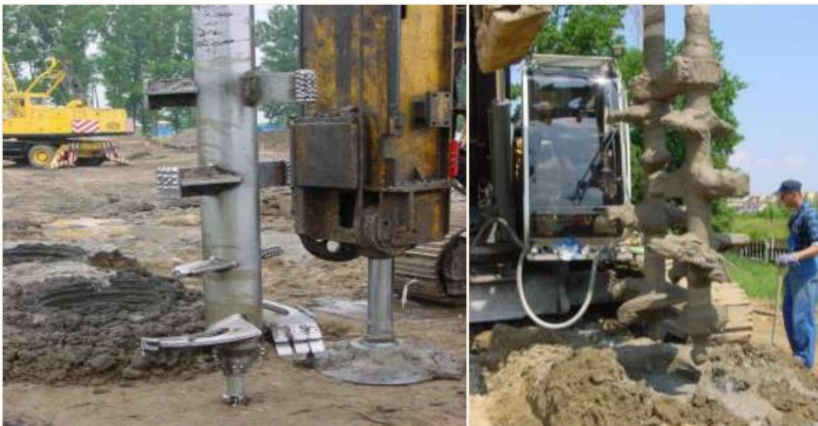
**Figure 2: Single and Multi-shaft mixing**
