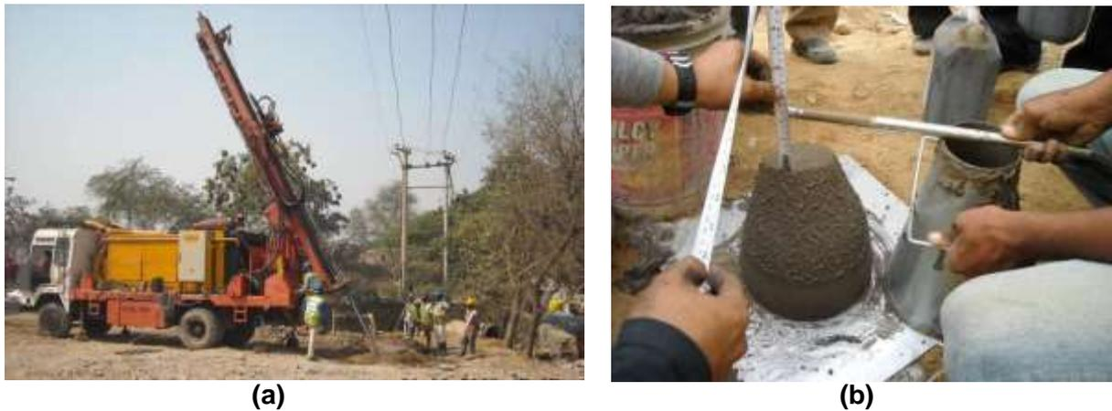
Fig. 10: a) Picture illustrating the progress of compaction grouting works at site b) Measurement of slump as QA-QC procedures
