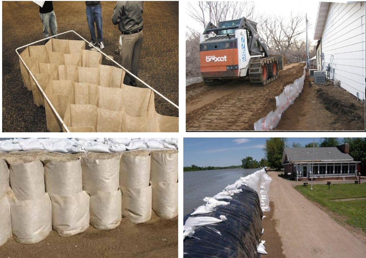
**Figure 34.** Geocell flood protection systems
