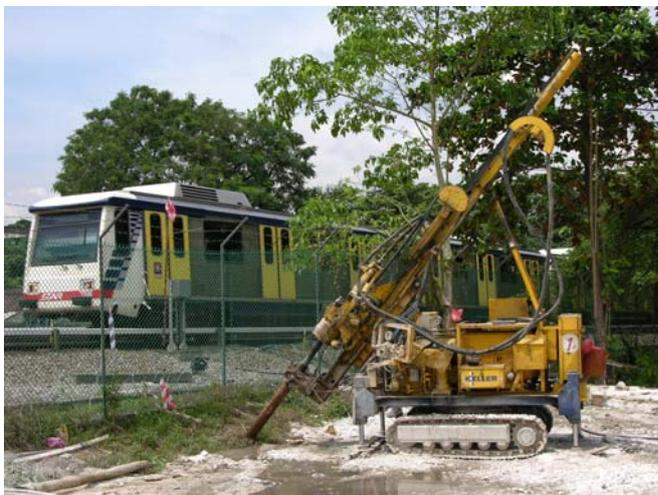
Figure 19 Grouting Beneath the “Live” Rail Track
