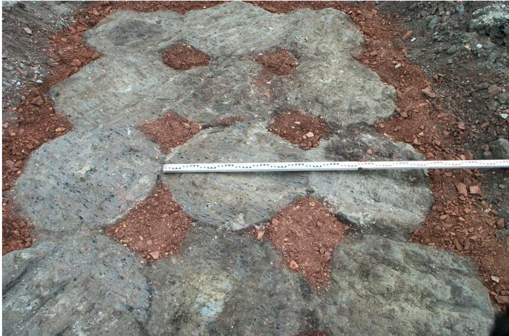
Fig. 2. Trimmed DSM columns at the bottom of a foundation pit
