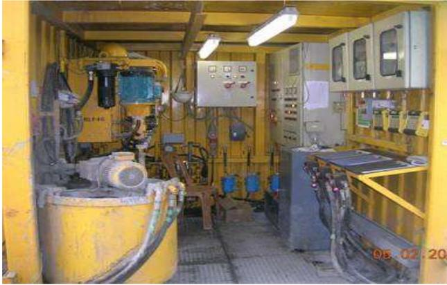
**Figure 7: Automatic Injection Containers – Computerised Grout Pumps**
