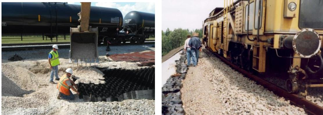
**Figure 6.** Geocells for constructing a rail road embankment on soft clay
