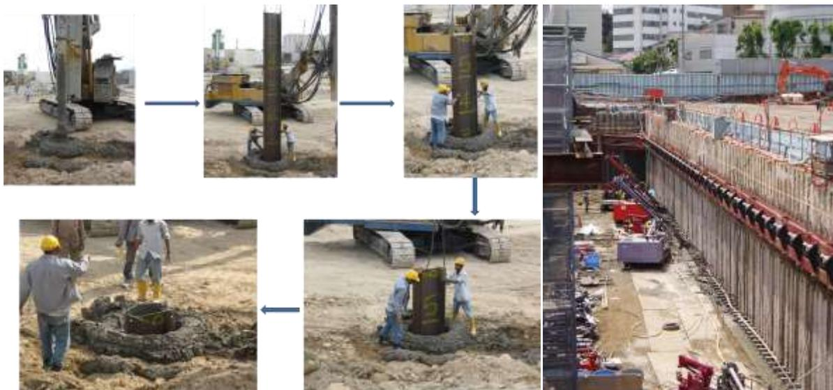
**Figure 10: Process of installing Steel H sections & Overall view of CDSM arrangements**
