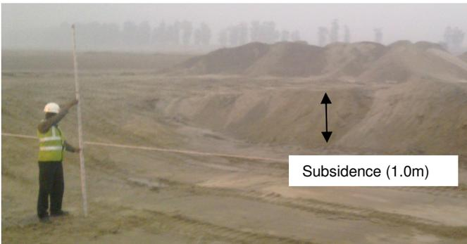
Fig. 7 The difference in levels achieved (about 1m) as a result of vibro compaction
