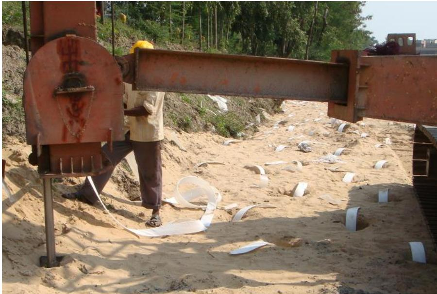
**Fig-2: Installation of PVD**
