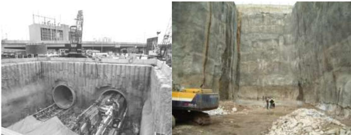
**Figure 21: NVM shaft & Dry walls after curtain grouting**
