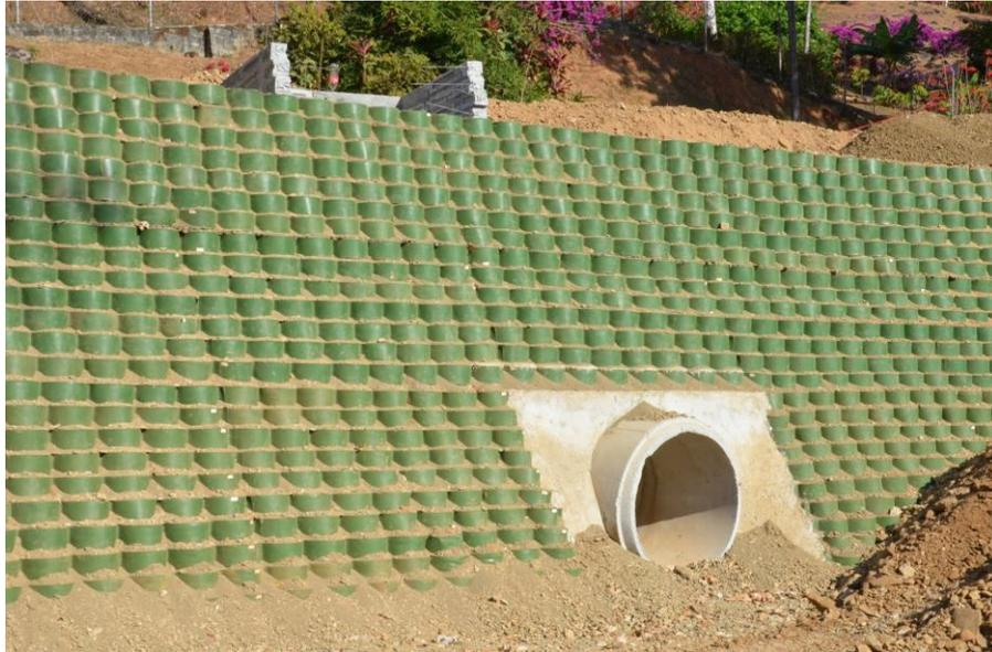
**Figure 18.** Finished geocell retaining wall
