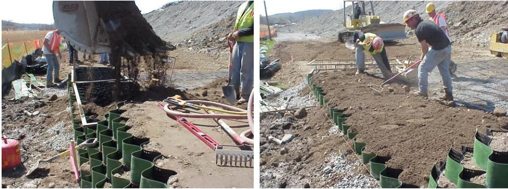
**Figure 4.** Filling of geocells
