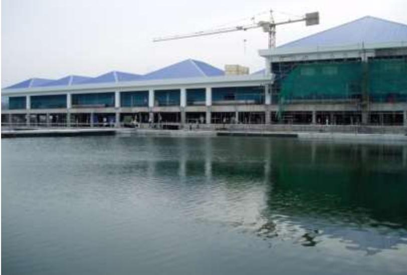
**Figure 18: Completed SBR tanks during hydro test**
