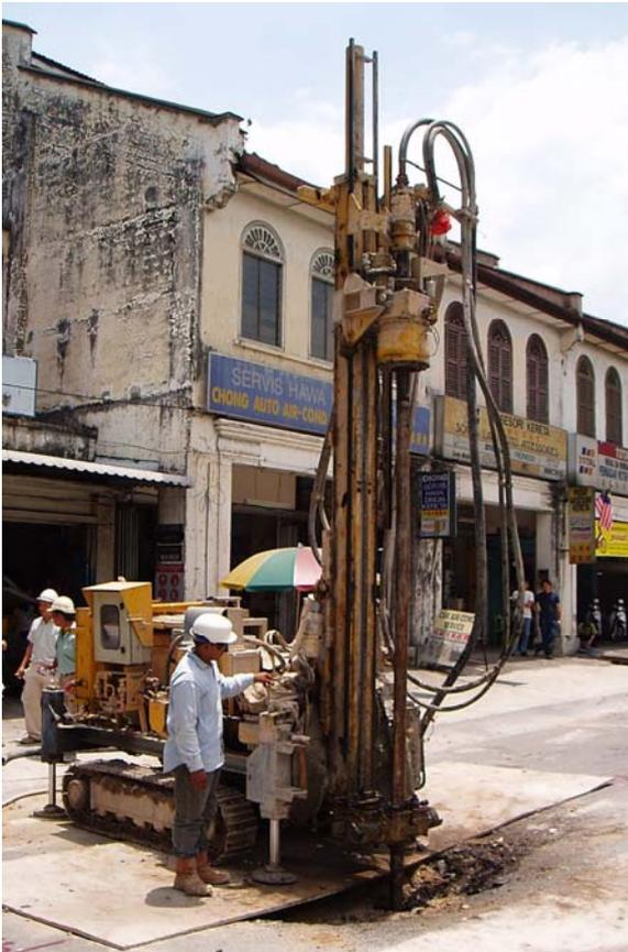
Figure 15: Treatment of Sinkhole and Ground Depression
