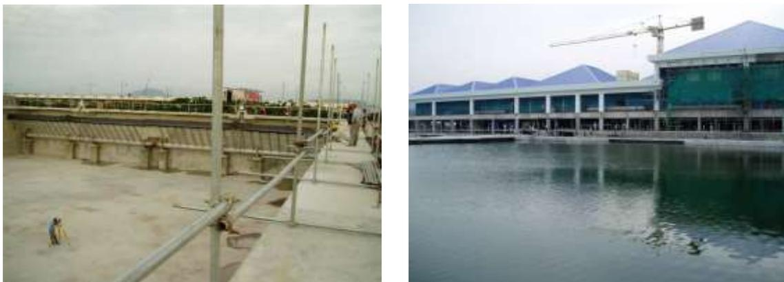
Figure 13. Completed SBR tanks – before and during Hydro test (Left: SBR 7&8 and Right: SBR 3&4 in the foreground and SBR 1&2 with 2 floors on top in the background).
