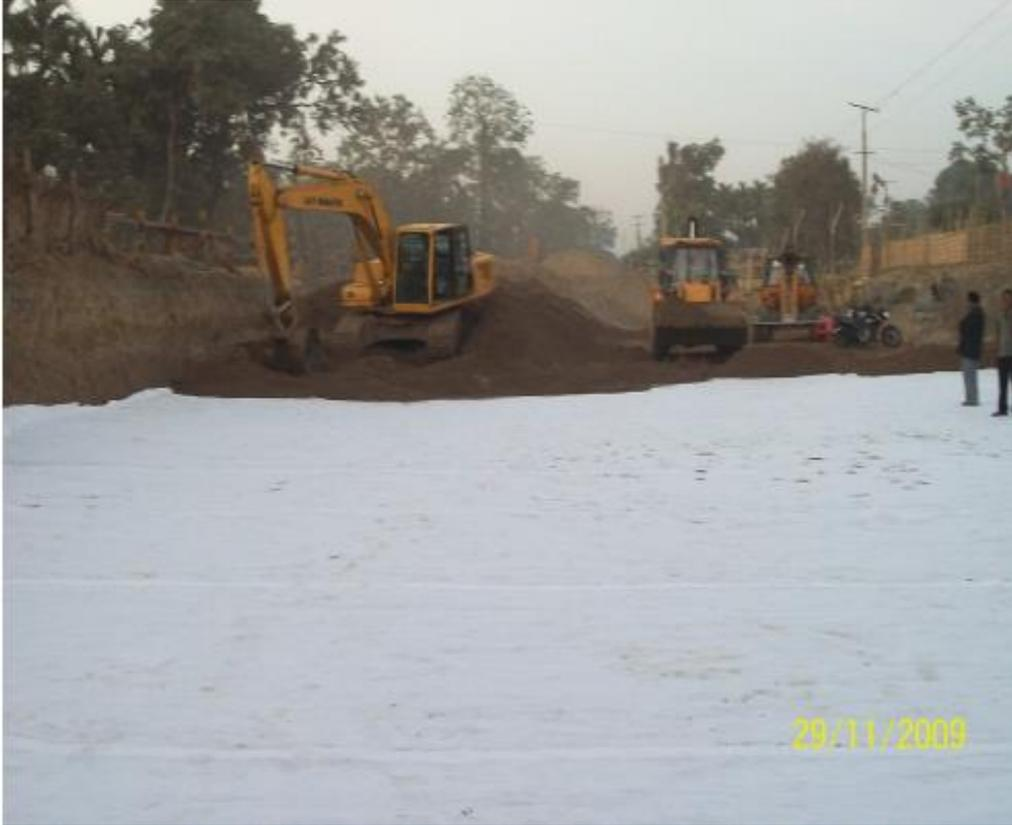
**Fig-3: Spreading of fill material over installed Geotextile**
