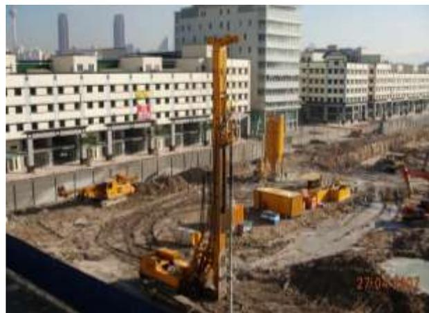
Figure 8. Execution of DSM works.
