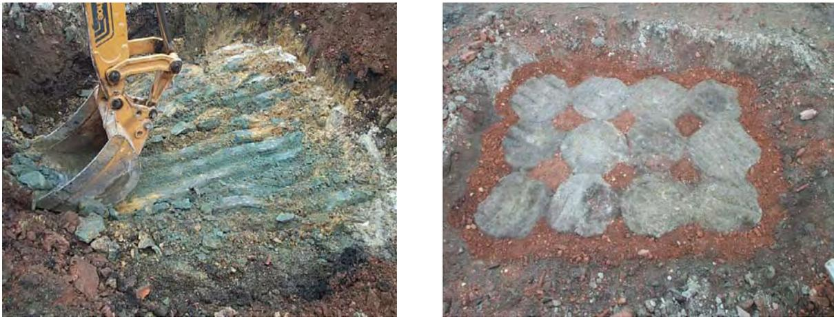
Figure 5. Exposed SM columns under pad foundation of a commercial centre (Megaplex, Katowice, Poland).
