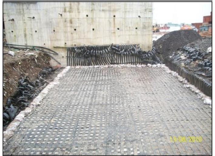
**Fig-3: Laying of basal reinforcement over pile caps**
