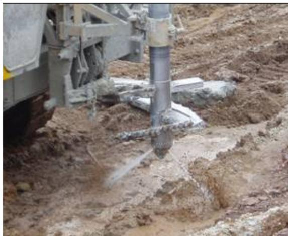
Fig. 12 Process of 'wet' DSM
