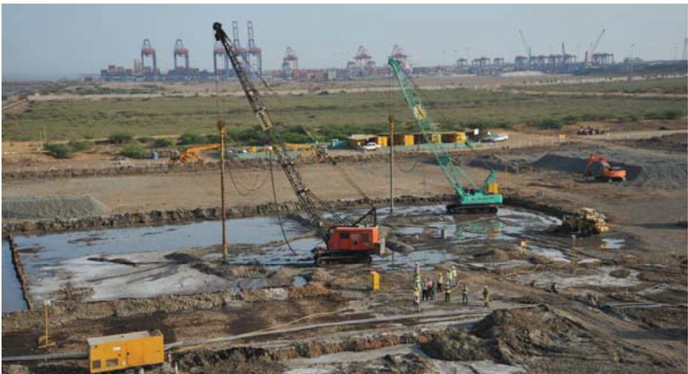
Fig. 6. Installation of Vibro stone columns by top feed wet method.
