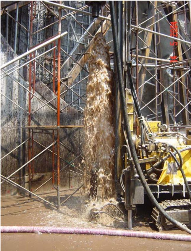
*Figure 17: Confined Water Inflow into Shaft During Grouting*
