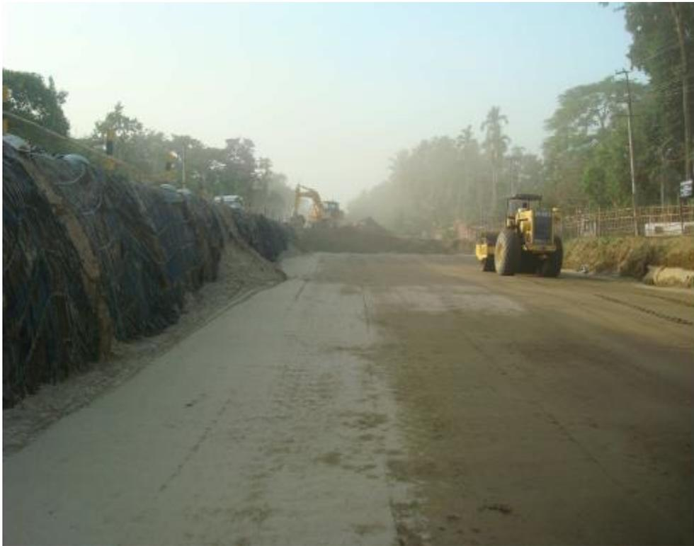
**Fig-4: Compaction of fill material over installed Geotextile**
