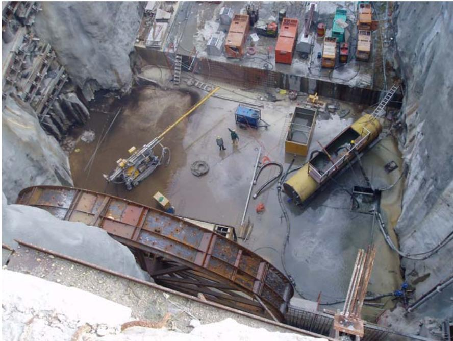
Figure 16: Location of Grouting Works at Launch Shaft
