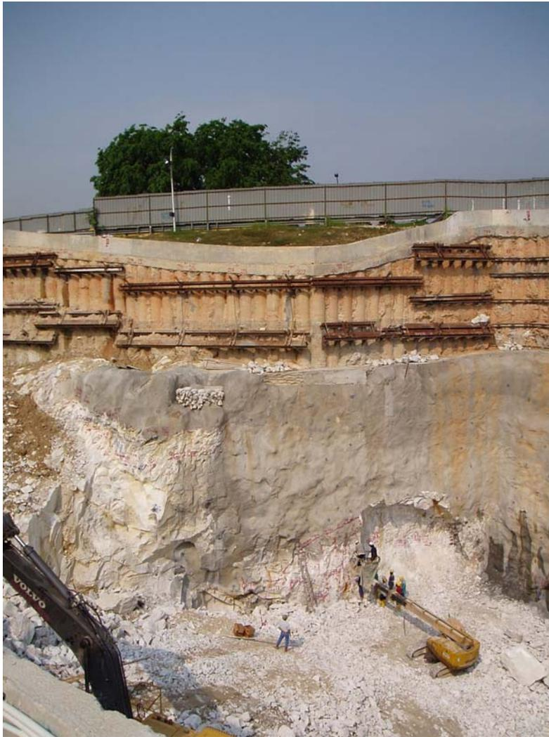
Figure 20: Dry Walls of Excavated Shaft
