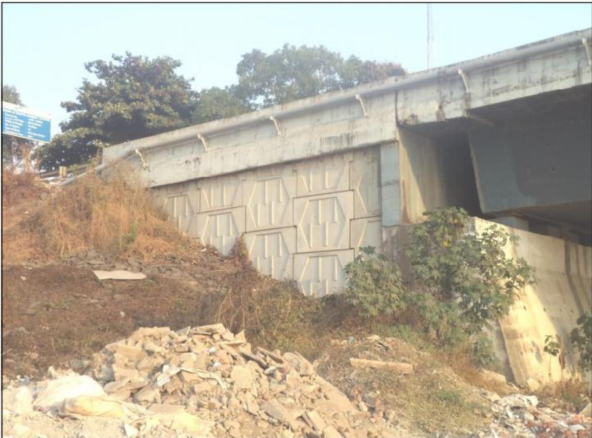
**Fig-4: Completed Reinforced soil wall structure**
