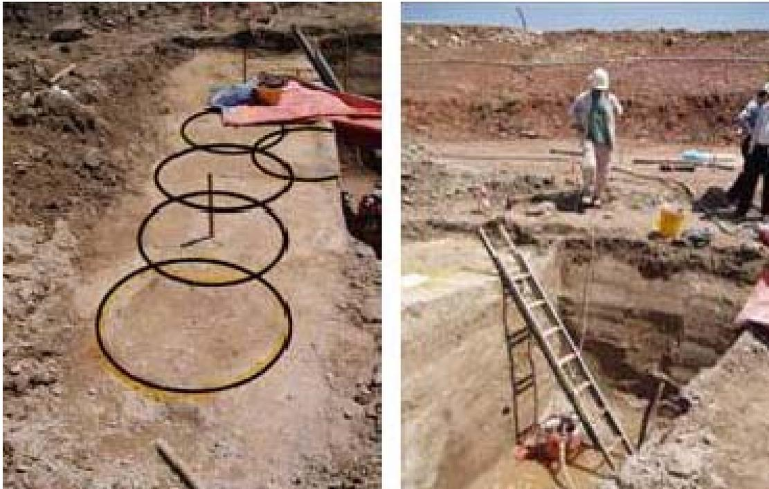
*Fig. 13. Exposed trial columns and subsequent excavation*
