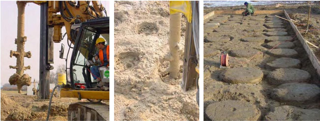
Figure 6. Soil mixing works and exposed columns for a bridge support foundation (A2 highway near Poznań, Poland).
