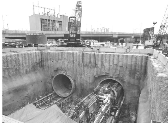
Figure 17 DSM Wall during and after TBM exit
