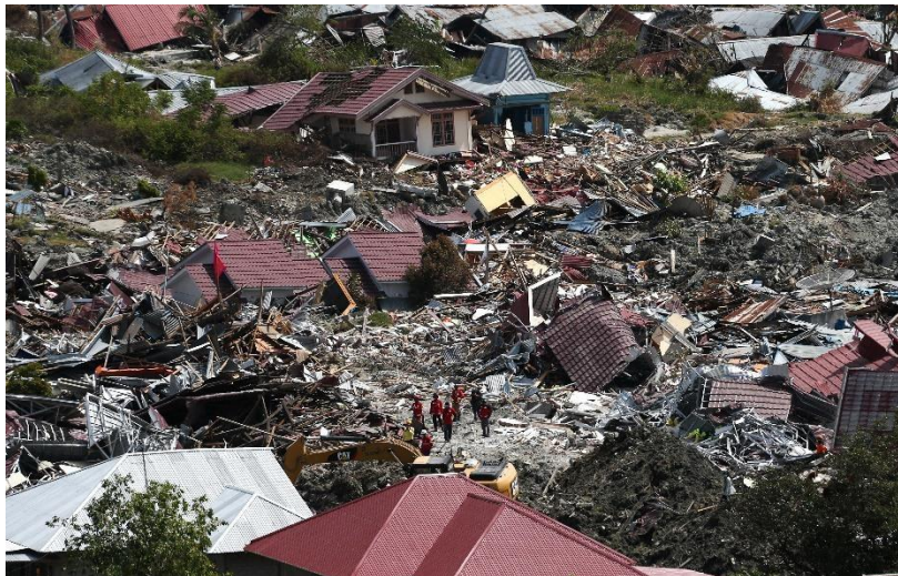
Fig. 3. Ground based image showing the destruction due to lateral spreading
