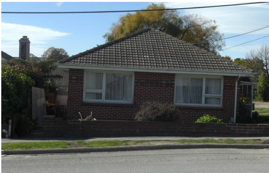
Fig. 1. Settlement and rotation of a residential structure following Christchurch earthquake of 2012
