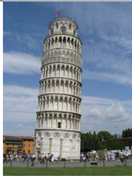
Fig. 1. Leaning of tower induced by different soil conditions under the foundation
