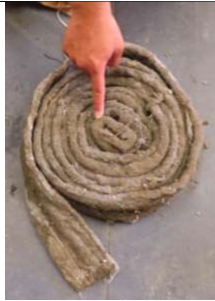
Fig. 2. Detected plastic drain that affected procedure of jet mixing.
