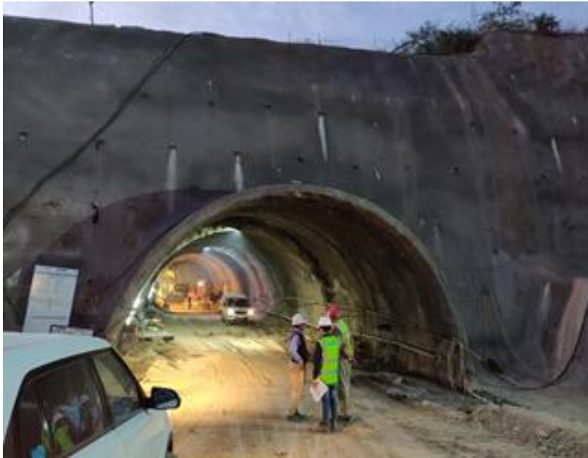
Fig.22 - Excavated heading of a tunnel in BBB railway project
