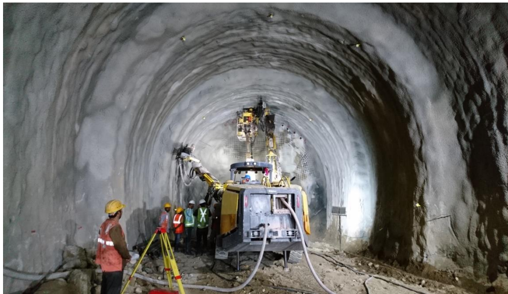
Fig.19 - Shotcrete application in Adit 3
