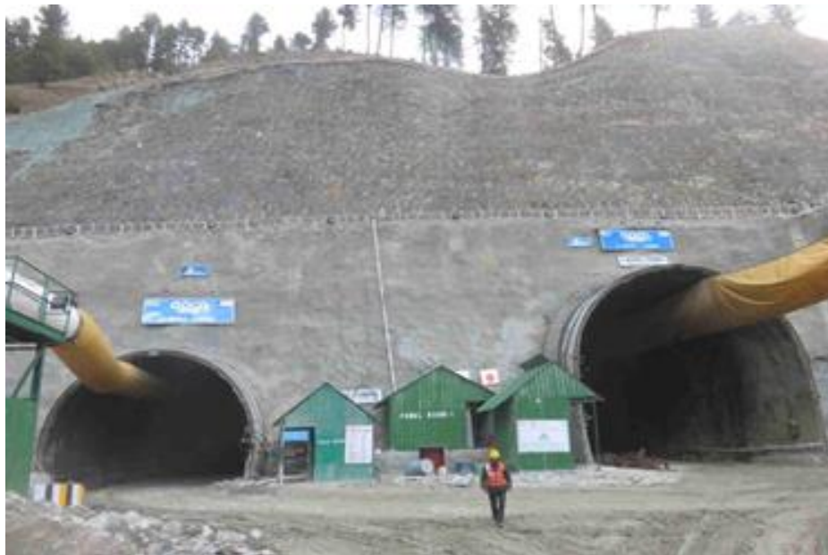
Fig.16 - Western portals of tunnels
