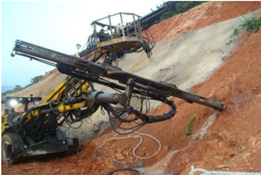
Fig.11 - Slope stabilization above rock cavern in Vishakhapatnam
