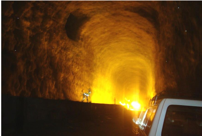
Fig.12 - Inside view of rock cavern for oil storage in Vishakhapatnam
