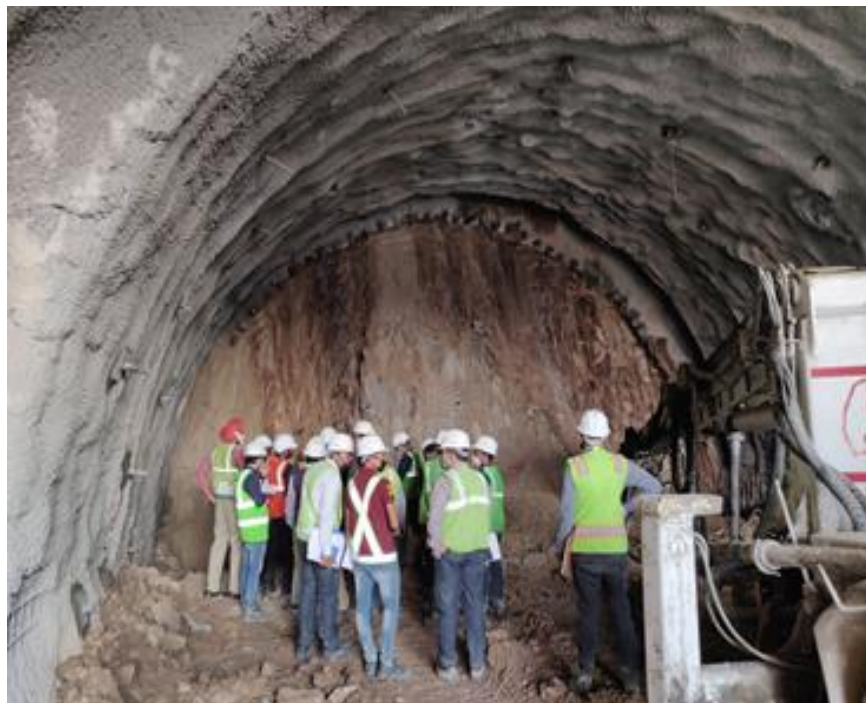
Fig.23 - Face geology of tunnel 1 in BBB railway project
