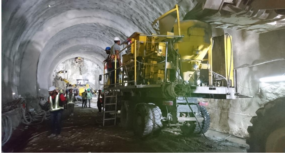
Fig.20 Blasthole drilling operation in Adit 3
