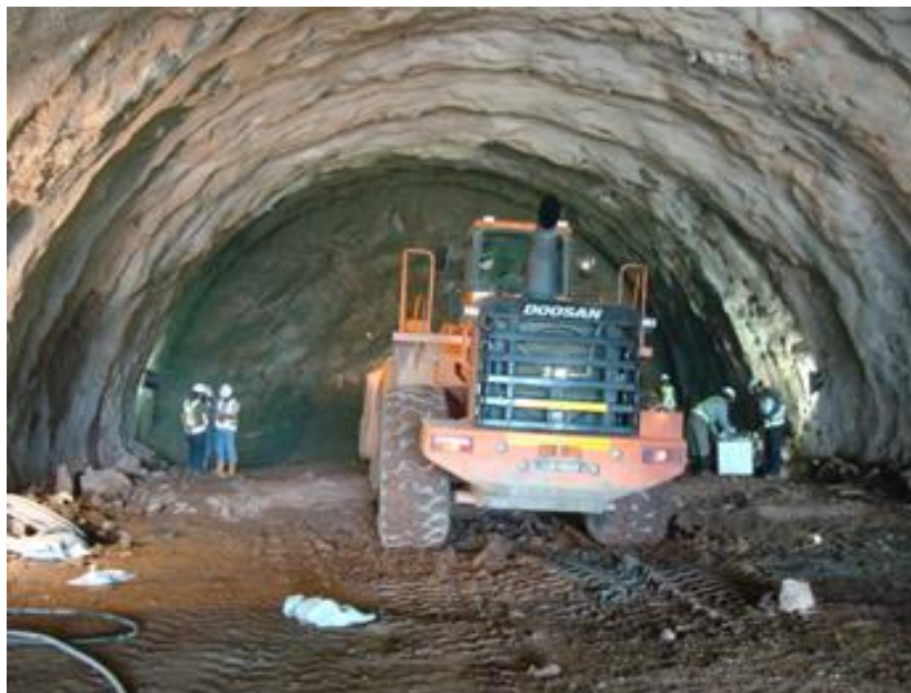
Fig.14 - Main tunnel view during excavation
