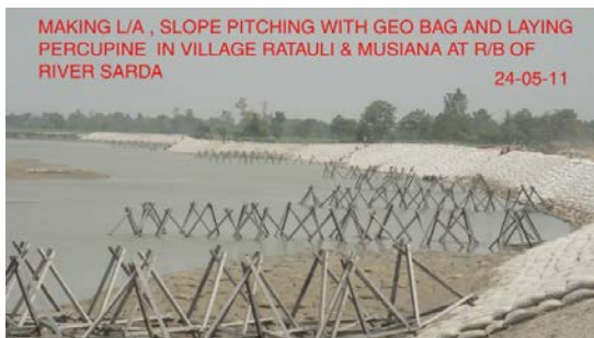
Fig.11 Use of sand bags (geocontainers) in erosion protection at River Sarada
