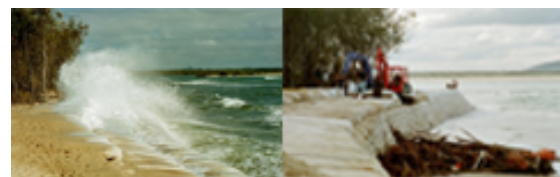
Fig. 10 Control Of Coastal Erosion By Geocontainers (Photo Courtesy : M.Venkataraman)
