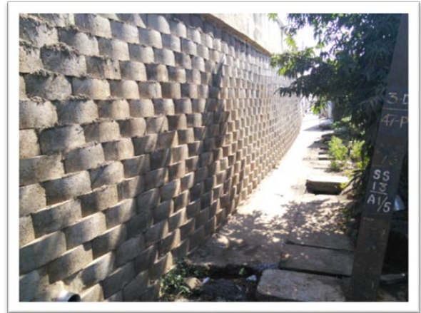
Fig.4 The Block faced wall at Eluru
