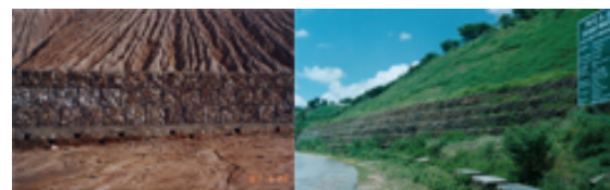
Fig. 9 Erosion control by Jute Geotextile in mine dumps (Photos courtesy Sri T.Sanyal)
