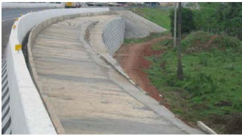
Fig. 8 The Bridge Approach at Siddhantam, A.P.
