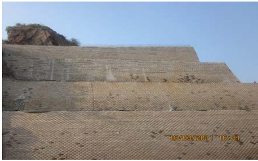
Fig.6 GRS Wall at Vijayawada
