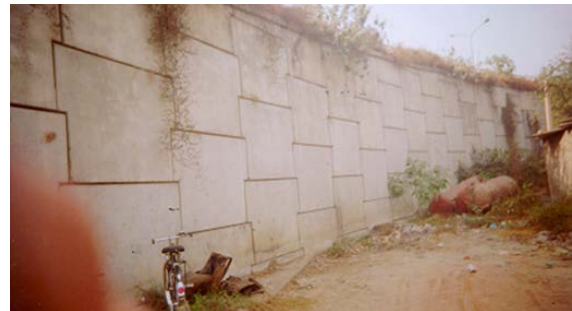
Fig. 1 First Reinforced Soil Wall in India – Ludhiana, Punjab 1986
