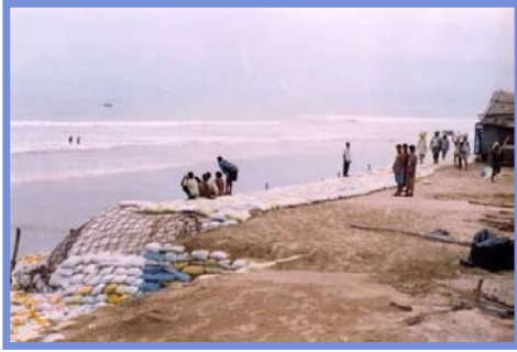
Fig. 12 Indigenous geotube for coastal erosion
