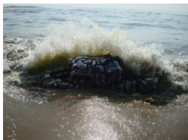
Fig. 2. Sand bag filled rope net gabions for shore line protection
