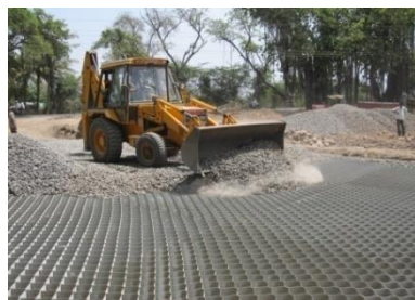
Fig. 3 Geocell reinforced road base on highly expansive soil
