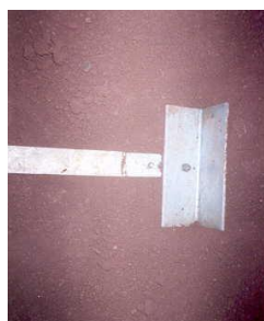
Fig. 6. Steel strips with end anchor
