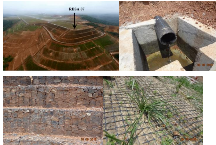
Figure 1. Some pictures from Kannur International Airport
