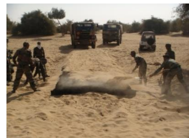
Fig. 4. Geocell reinforced road in desert by Indian army
